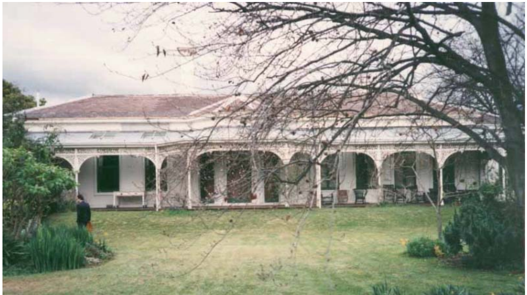
Figure 17. Front façade of ‘Tintern’ with a canted bay at its centre. The verandah iron is c1870s. (source: National Trust, n.d.)
