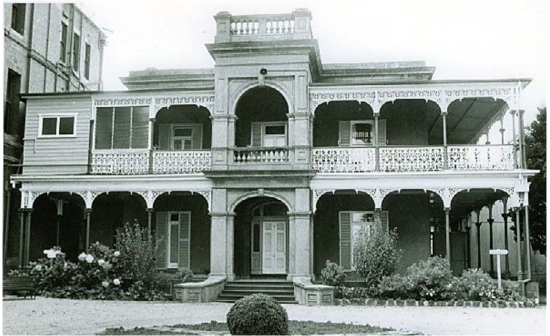
Figure 13. 'Bryn Mawr', 172 Burke Road, Glen Iris (HO7). Built in 1859 to a design by architect George Wharton, two-storey balcony and rendered portico added in the 1870s. (source: National Trust, nd)
