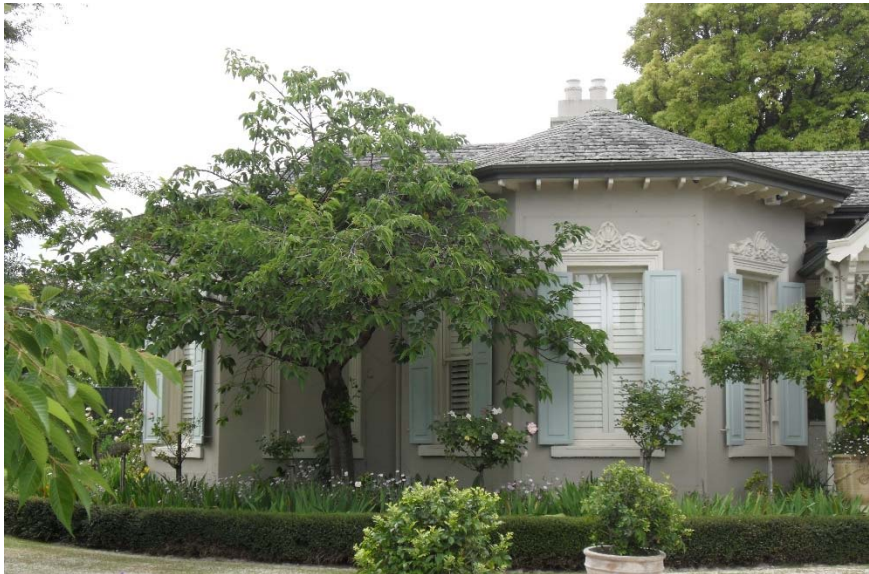
Figure 11. The semi-hexagonal bays at the north end of the house. (source: Context, 2016)
