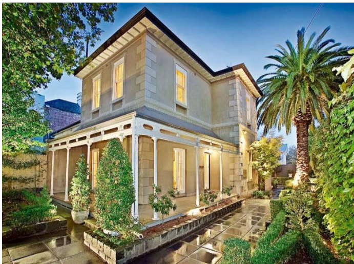
Figure 16. 'Shipley Lodge', 76 Caroline Street with its wide eaves and simple modillions. (source: realestate.com.au)
