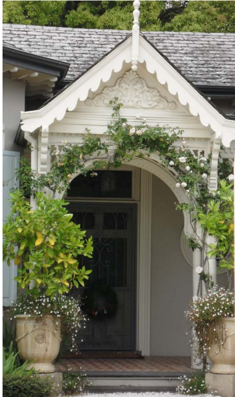
Figure 12. Detail of the gabled entrance portico. (source: Context, 2016)
