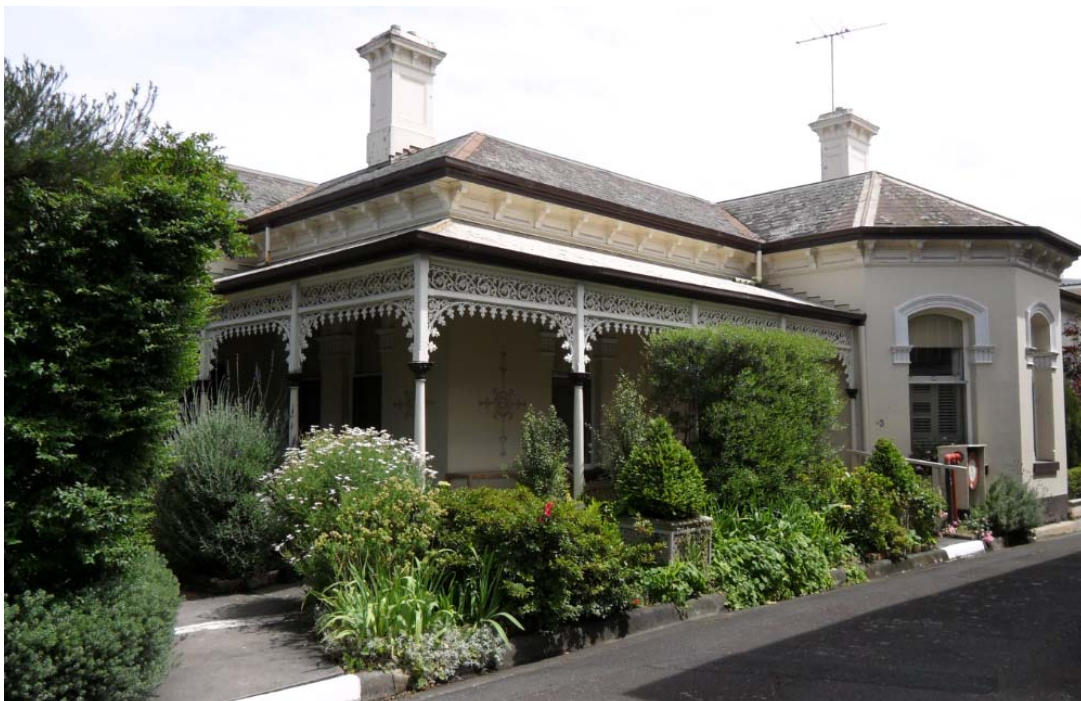
Figure 5. View of the east side elevation and part of the front (left), showing the slated hipped roof, bracketed chimneys and eaves, cast-iron verandah detail, and label moulds to the segmentally arched windows of the semi-hexagonal bay. (source: Context, 2016)
