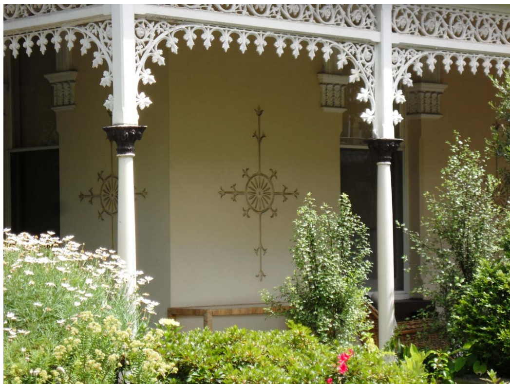
Figure 6. Detail of the cement render ornament below the verandah. (source: Context, 2016)
