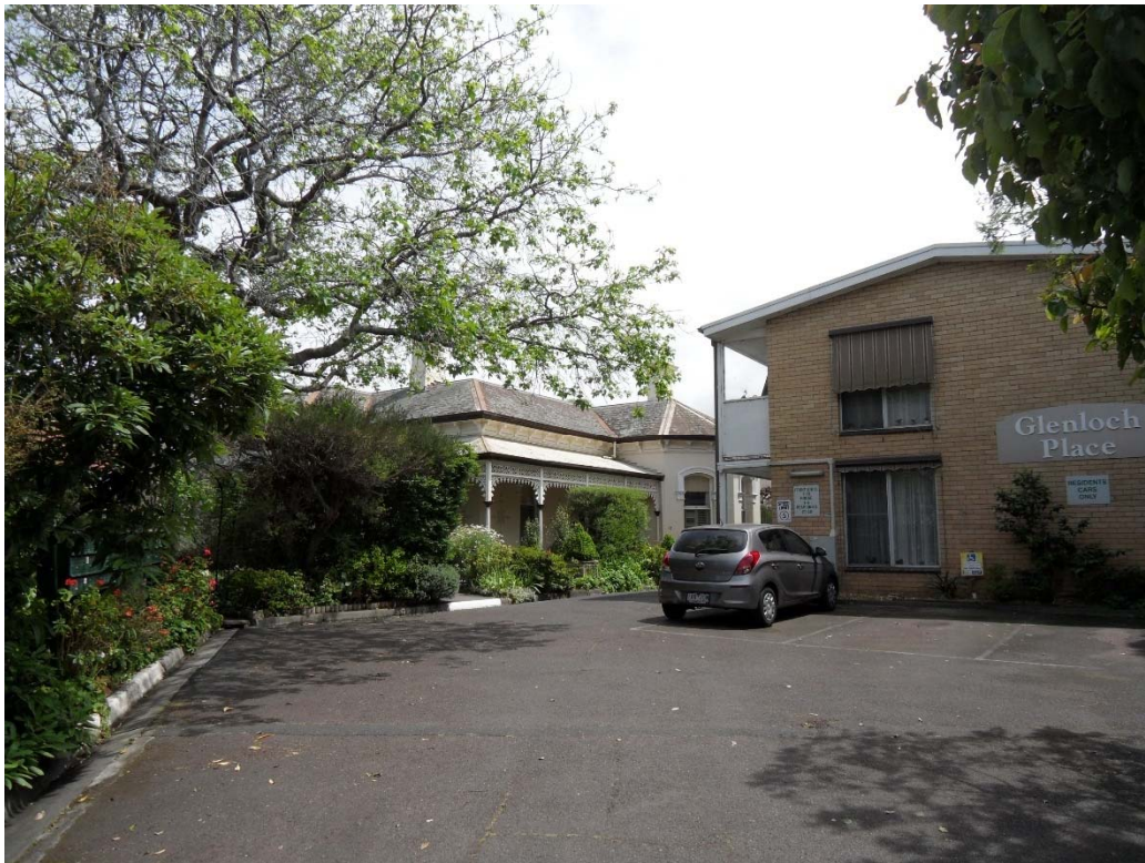
Figure 4. View of 'Cullean' with the post-war flats beside it. (source: Context, 2016)
