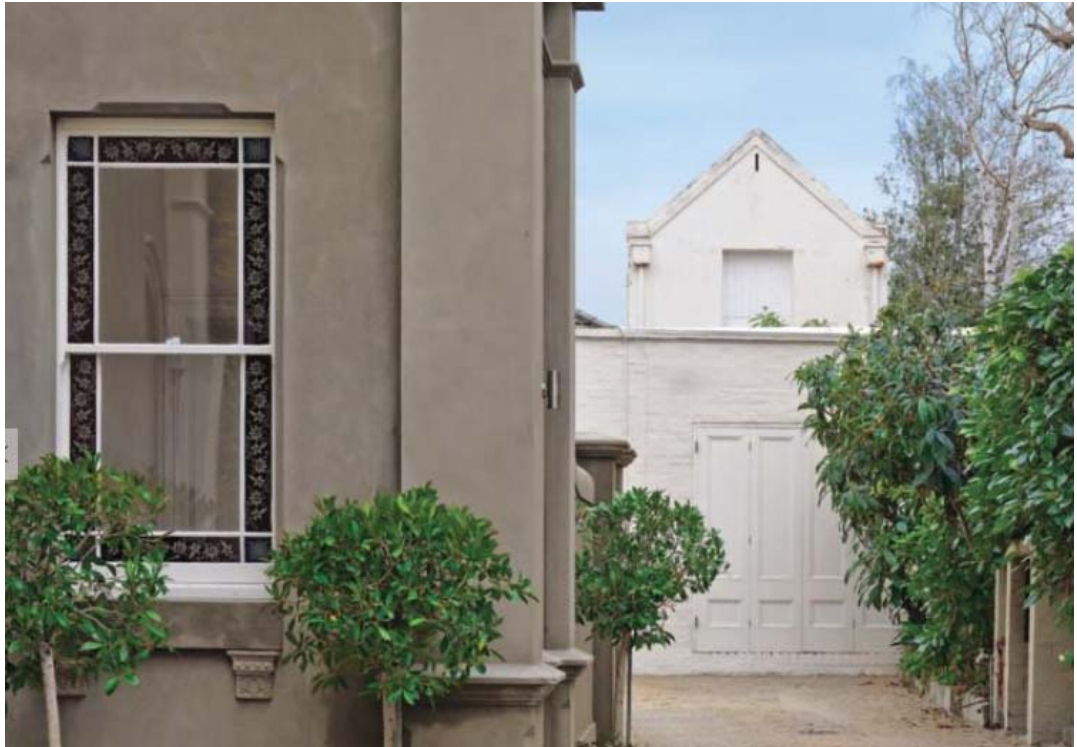
Figure 3. The side of the house and the western (front) elevation of the former stables (source: Abercromby's Real Estate, 2011).
