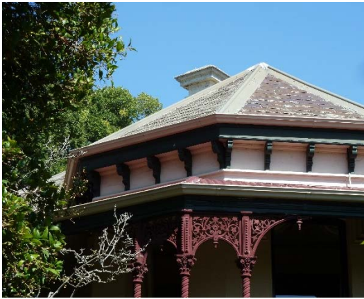
Figure 665. Detail of hipped roof to canted bay and eaves brackets (source: Context 2016).
