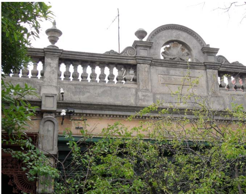
Figure 2. Detail of the parapet of no. 64 (and part no. 66), showing the ochre-yellow limewash to the render. (source: Context 2016)
