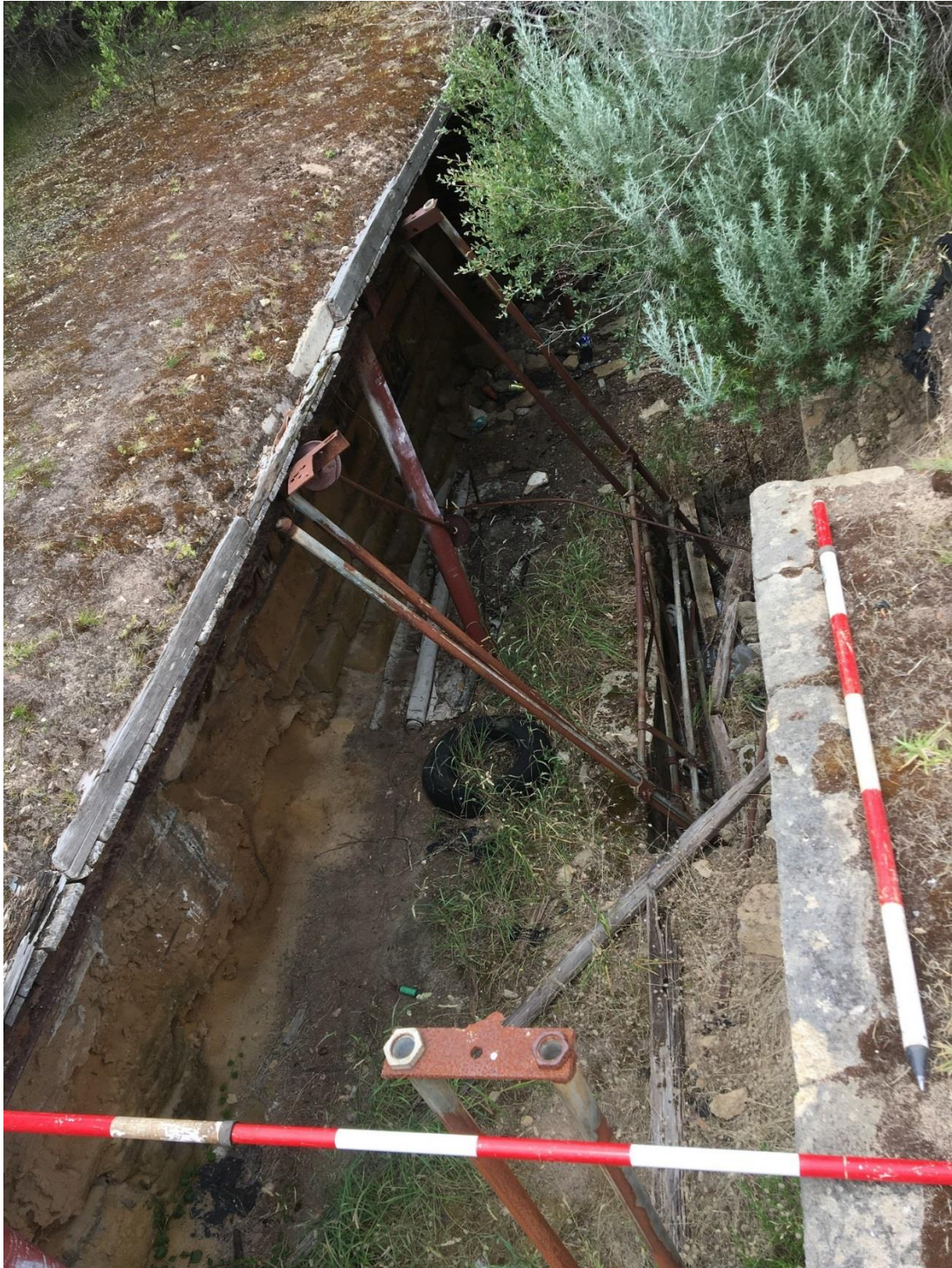
Figure 10 Constructed trench at forward (northern) face of rifle butts. Timber and masonry construction material visible. Steel components of target frames and pulley system evident. Rolled rifle targets are also visible at base of trench.
