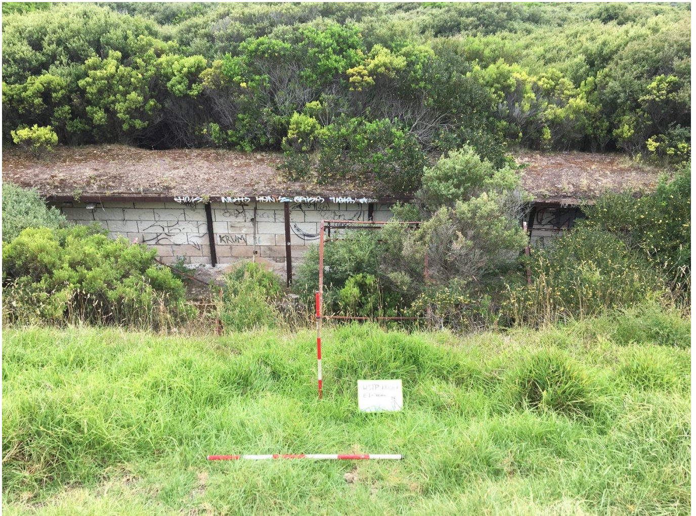
Figure 15 Eastern section of trench appears to be of newer construction. Materials used include masonry and reused railway track. Steel target frame visible in centre of shot.
