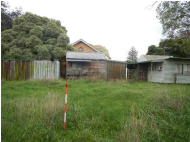
Southeast of site facing northwest towards extant dwelling and sheds
