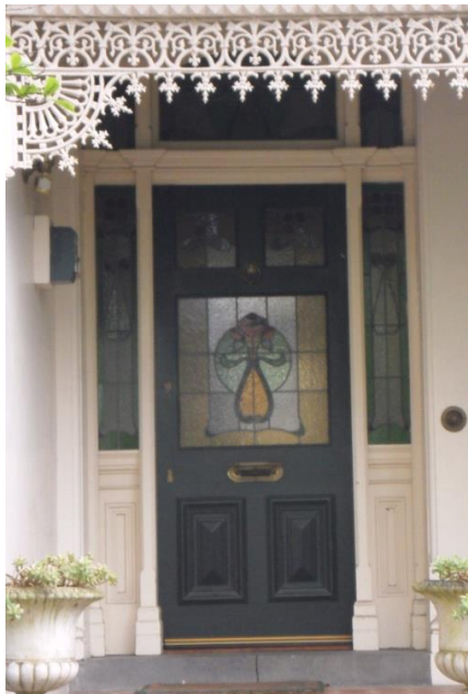
Figure 5. Early twentieth-century door and leadlights at 5 Avondale Road. (source: Context, 2017)
