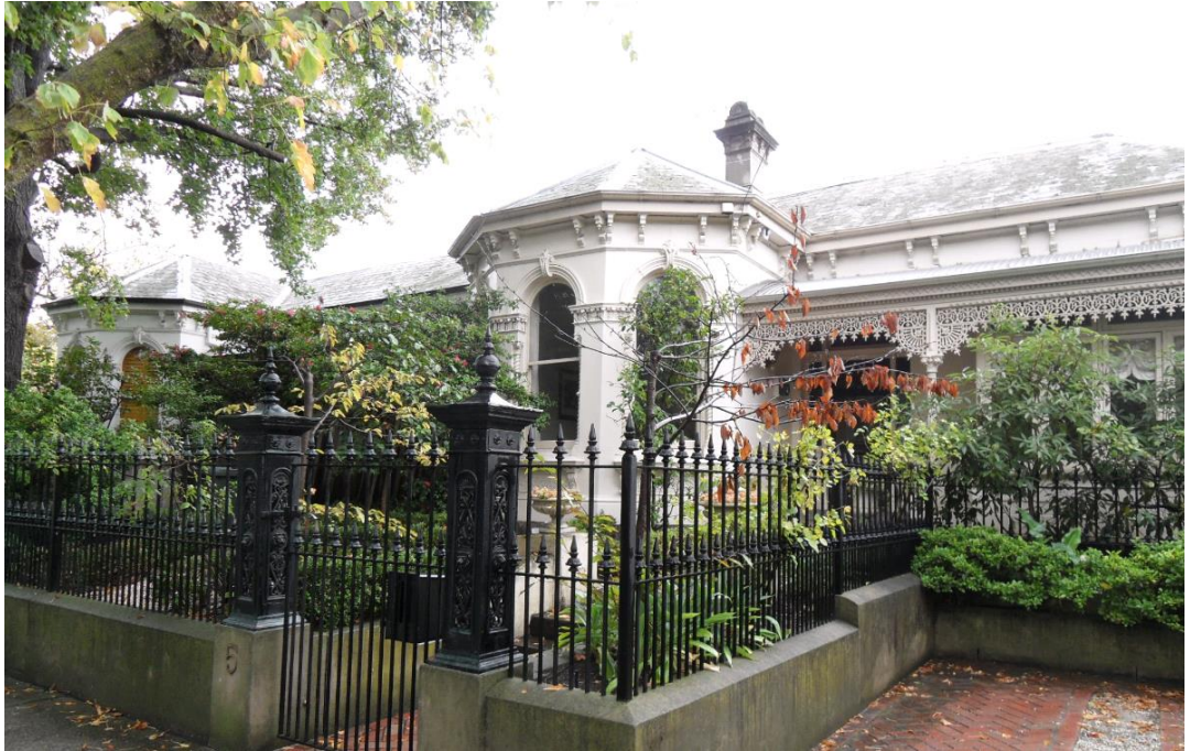
Villas at 3 (left) and 5 (right) Avondale Road.
