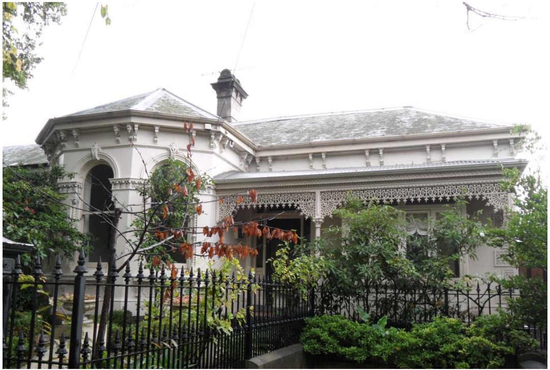
Figure 4. Front façade of 5 Avondale Road. Note casement box bay window beneath verandah. (Source: Context, 2017)
