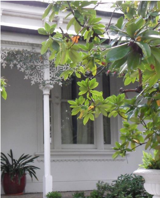
Figure 6. Original front window at 3 Avondale Road with dogtooth moulding below sill. (Source: Context, 2017)
