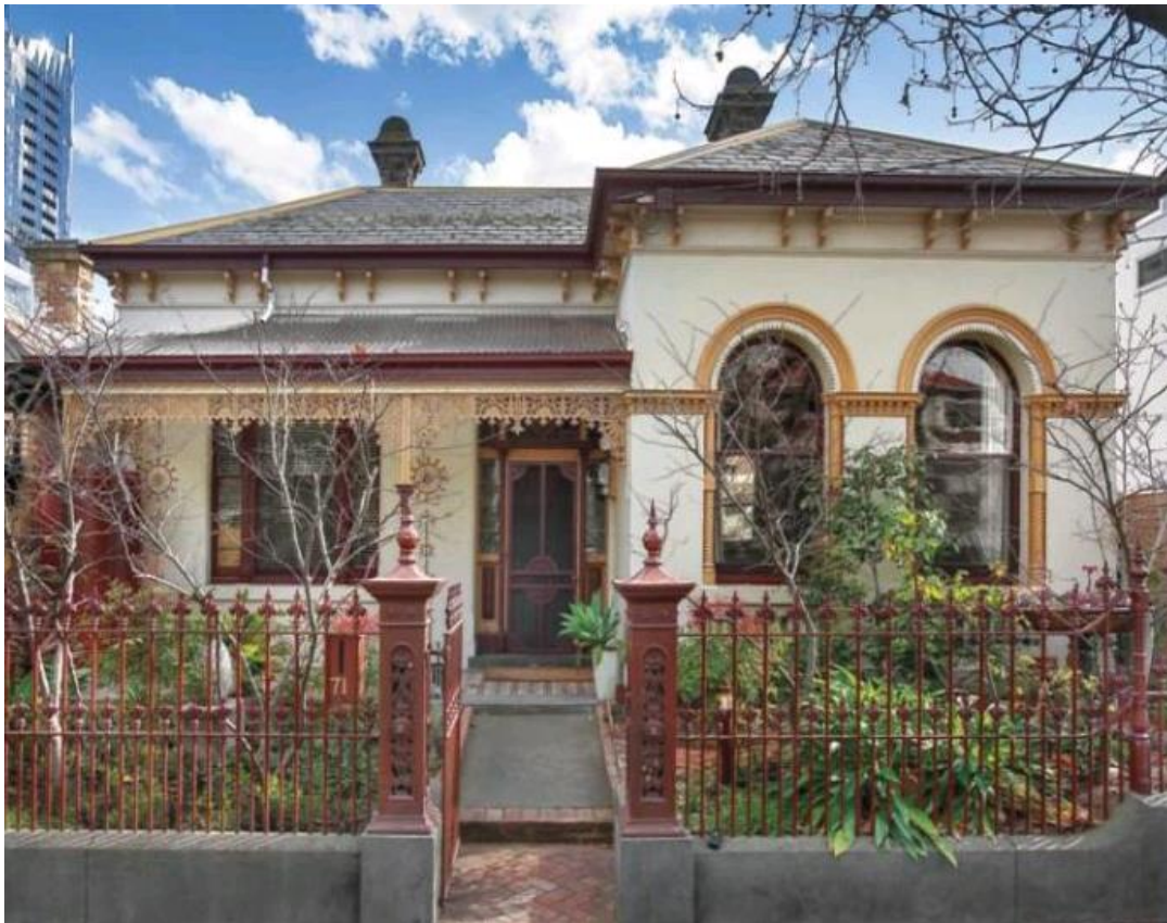
Figure 9. 71 Tivoli Road, South Yarra (Significant in HO149). (Source: Abercrombies, 2013)
