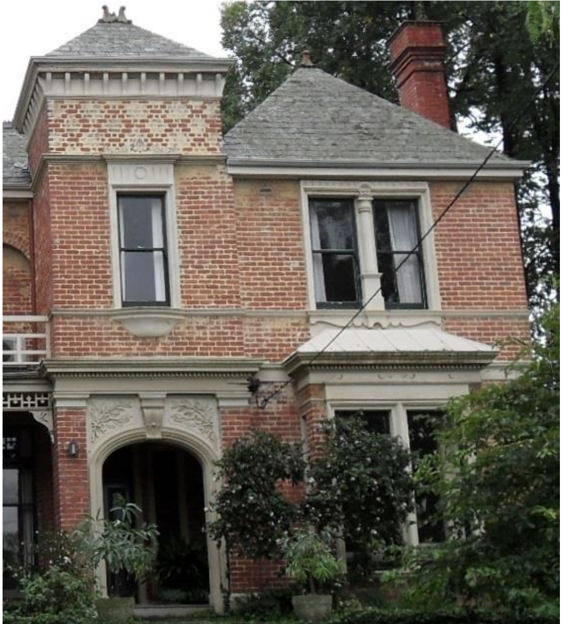
Figure 7. Classically inspired cast-cement surrounds to the window and door openings. (Source: Context, 2017)
