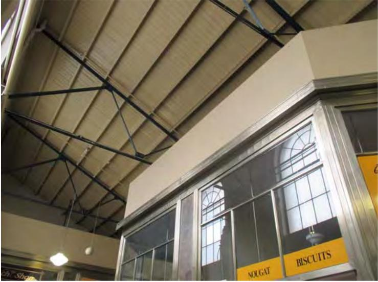
Figure 6 Original roof trusses and lining boards to Dairy Produce Hall; fall arrestors above the stalls were constructed recently
