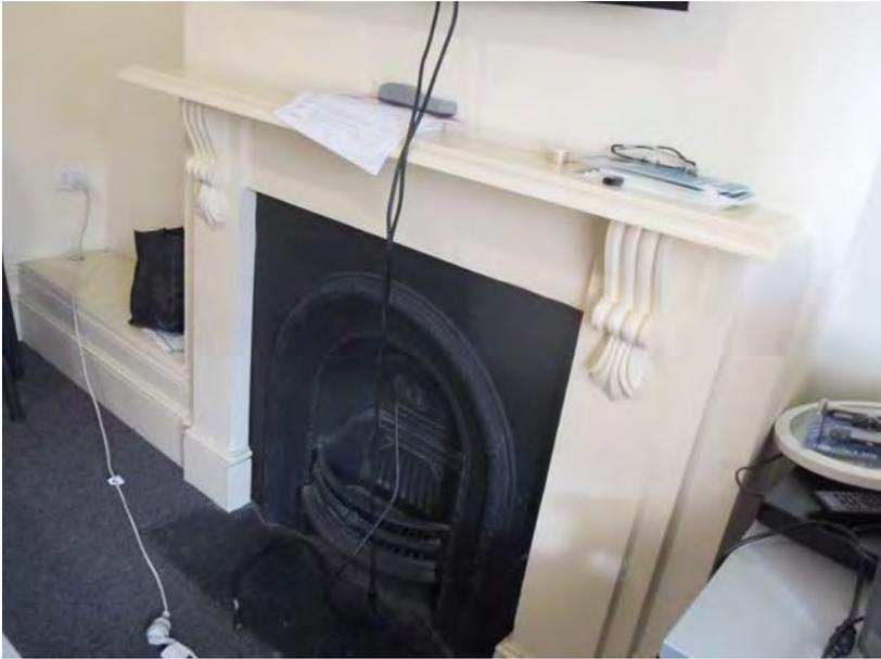
Figure 4 Early fire place at first floor level
