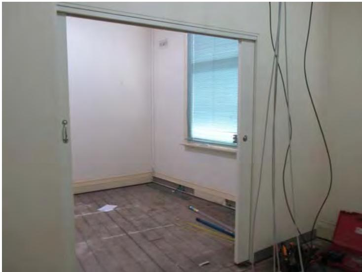
Figure 4 New openings between terraces
