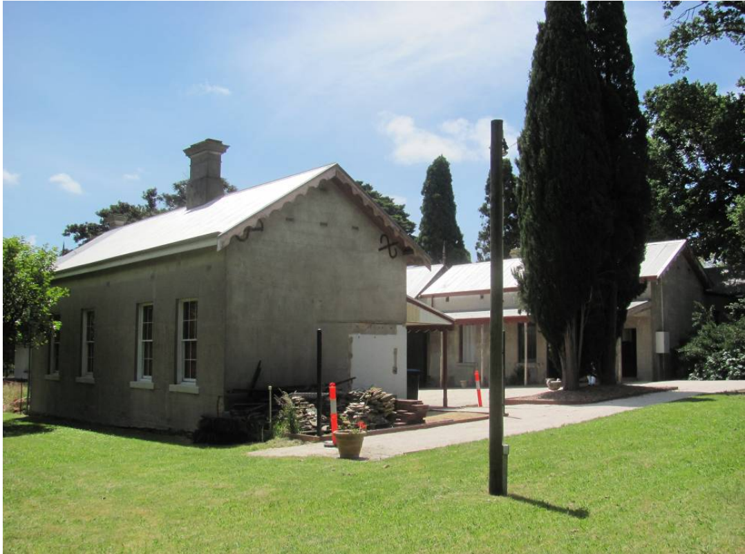
Figure 9 - View from the southwest showing the two courtyard wings and the pair of Italian cypresses. The white patch on the facing wall shows the previous location of the now demolished WC (Source: Context 2012)
