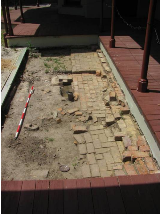
Figure 25 - Recently excavated area to the north of the house, showing the brick platform with additional courses of brick to support the veranda. (Source: Context 2012)
