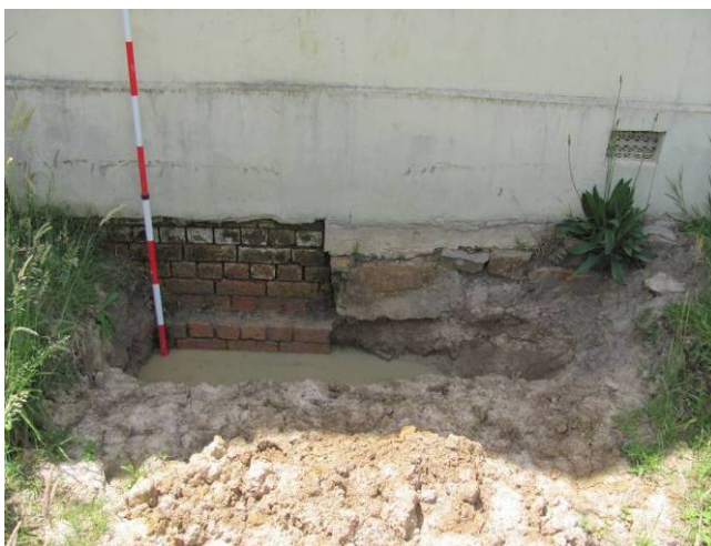
Figure 5 - Trench excavated against the south-western wall of the main house, showing the different foundations beneath Rooms 10 (left) and 11 (right). (Source: Context 2012)
