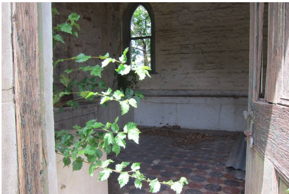
Figure 24 - Cool store or dairy showing tiled floor and masonry benches. One of two pointed arch headed windows is visible in the background. (Source: Context 2012)
