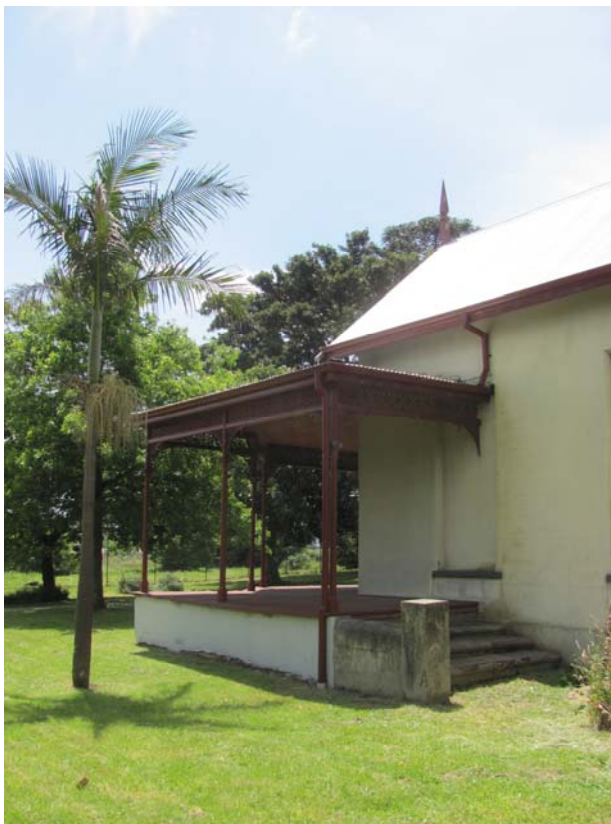
Figure 7 – The west end of the veranda colliding with one of two blind windows (the other is to the right) (Source: Context 2012)
