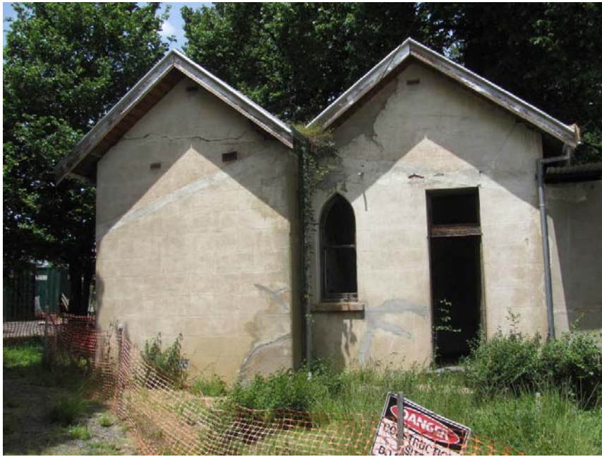
Figure 11 - Outbuilding with store rooms to the left and cool store or dairy on the right. The laundry is at the extreme right of the photo. The evidence of the roofline of a former building is clearly marked in the render surface. (Source: Context 2012)
