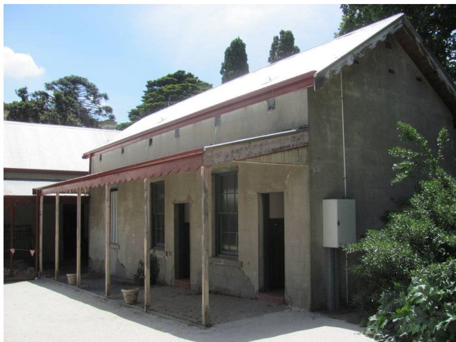
Figure 10 - South eastern courtyard wing as viewed from the courtyard. The veranda has been reconstructed. (Source: Context 2012)
