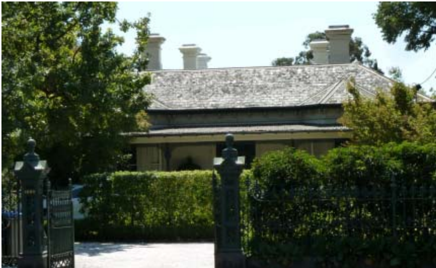
Figure 8. 'Lillirie' at 1089 Malvern Road, Armadale, individually significant HO273 (source: Context 2016).
