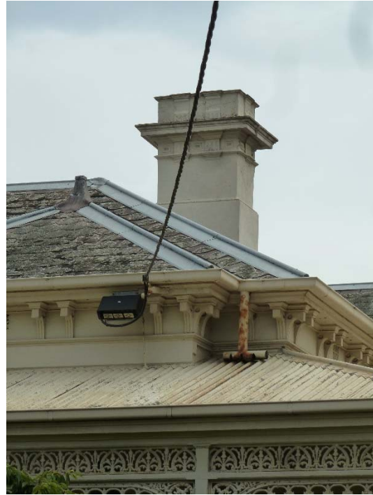
Figure 7. Detail of chimney and eaves (Context 2016).
