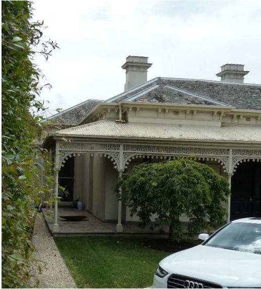
Figure 6. View of return verandah to the west elevation (source: Context 2016).
