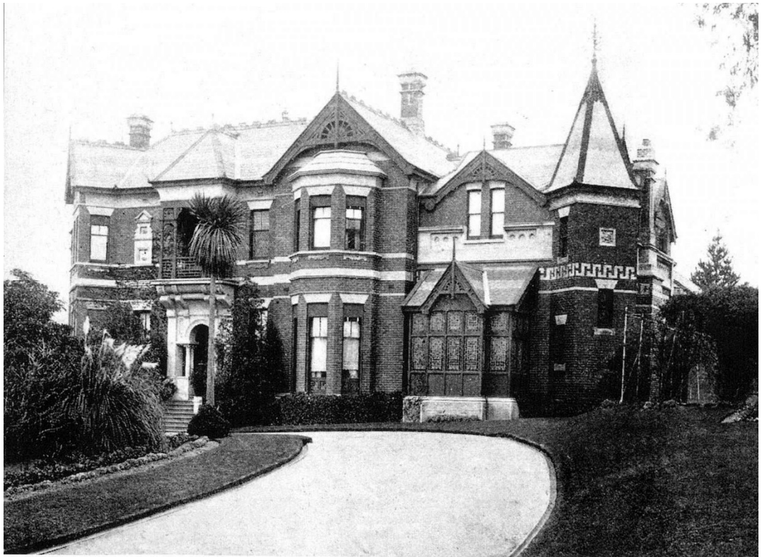
Figure 7. 'Homeden' on Lansell Road, Toorak (demolished). Designed by Reed, Henderson & Smart, 1889. (source: Lewis 2004:80)
