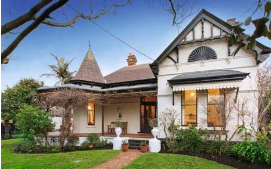
Figure 6. 15 Forster Avenue, Malvern East, of 1890 (HO310). (source: Marshall White, 2015)
