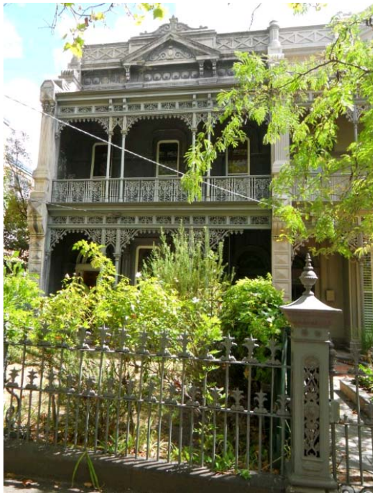
Figure 3. 13 Cromwell Road, South Yarra (H10228) (source: Google Streetview).
