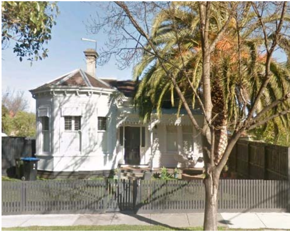
Figure 3. 59 Northcote Road, Armadale (Significant in HO130). (source: Google Streetview)
