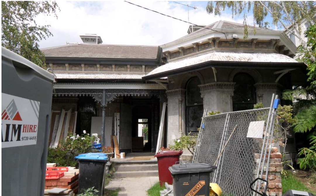
Figure 2. 30 Lewisham Road, Windsor, while undergoing work in 2016. (source: Context 2016).
