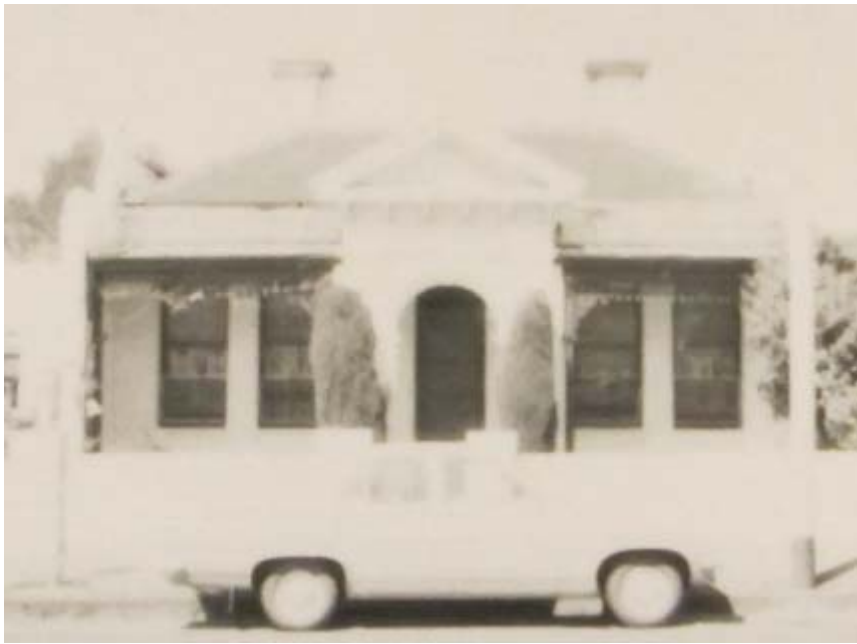
Figure 3. 36 High Street during the 1970s before the current front wall was built. (source: CUA collection, SLV).
