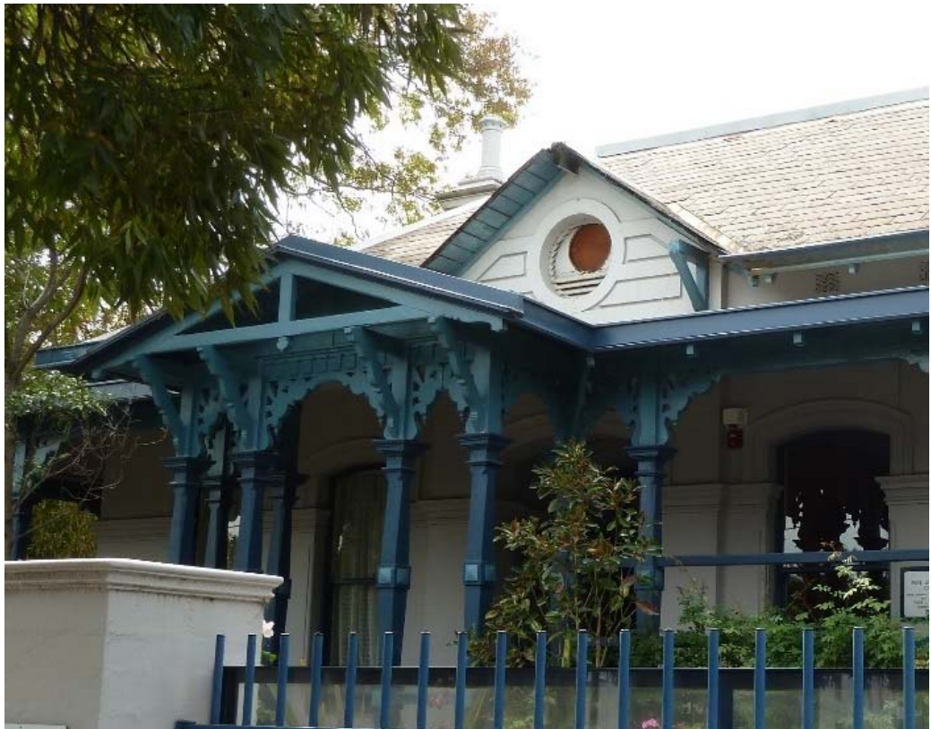
Figure 4. Detail of front veranda gable and unusual timber brackets (source: Context 2016).
