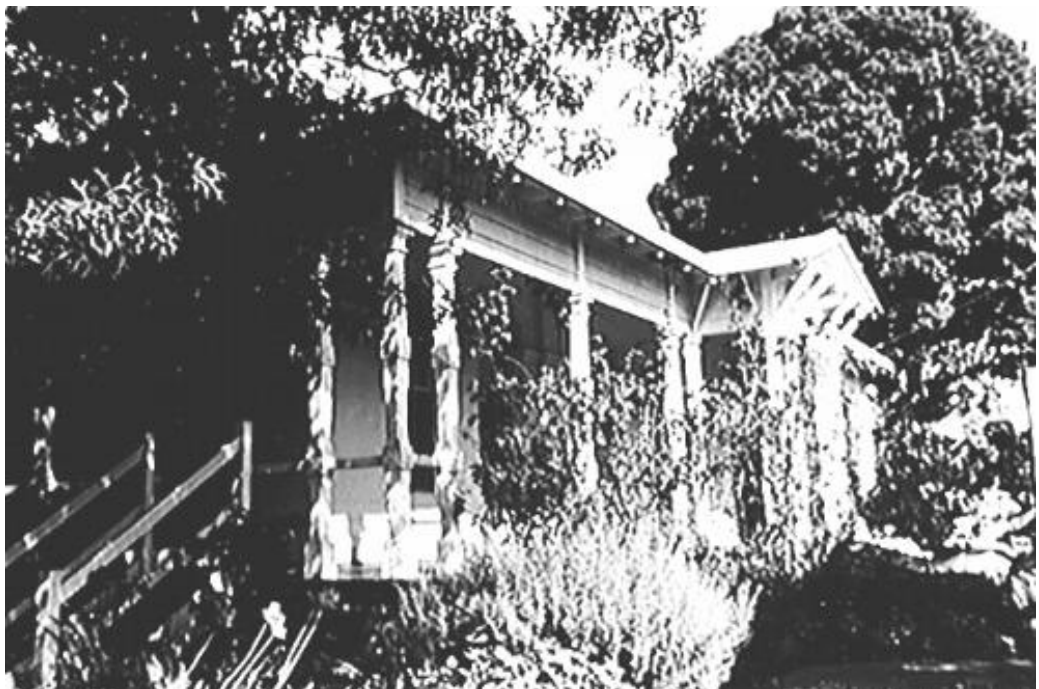
Figure 2. Photograph of the façade of 20 Wallace Avenue, from the north, 1984 (source: Malone 1984).
