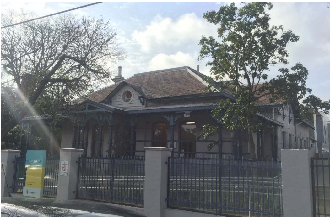
Figure 5. View looking north-east showing the southern side gable (source: City of Stonnington 2016).
