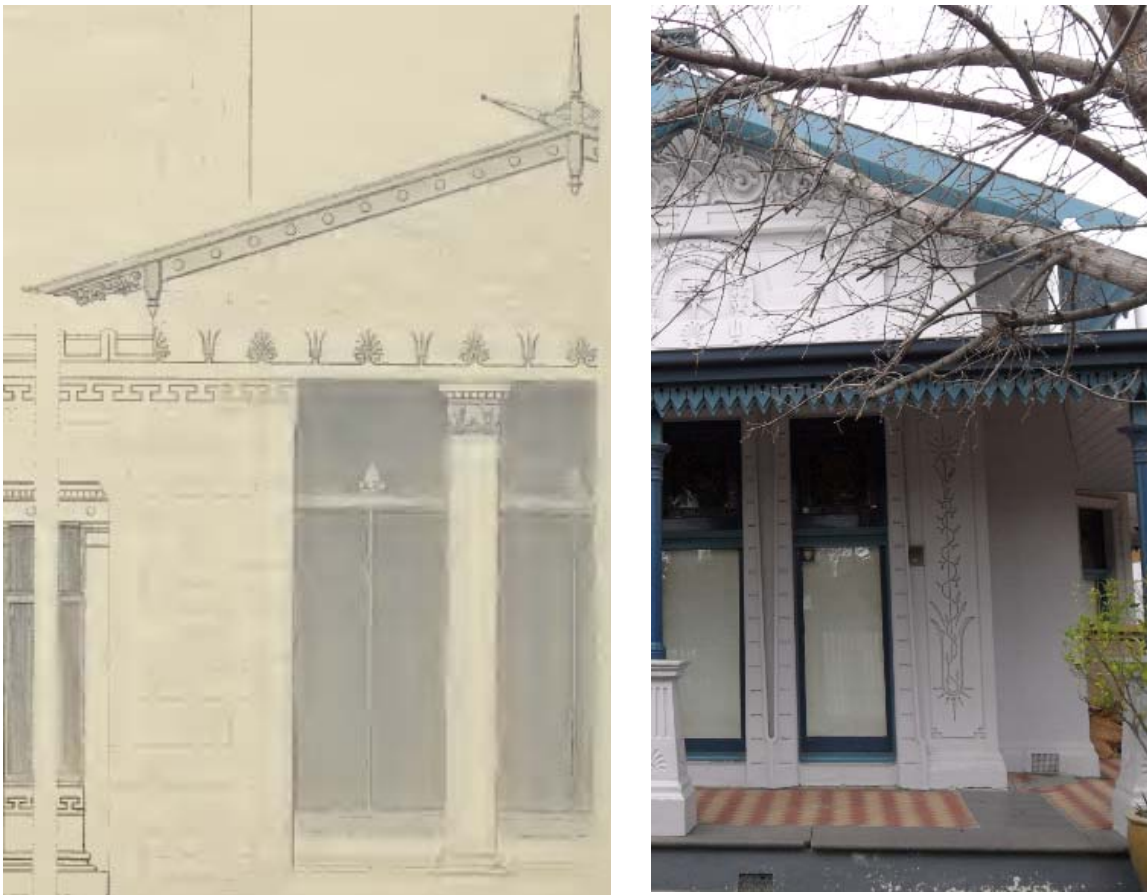
Figure 12. Front gables of 'Holmwood' (left) and 'Hybla' (right). Note low pitch of gable, metal bosses along bargeboard, scrolled ends of bargeboard. The incised patterns below the gable of 'Hybla' are shown more clearly below (source: Blackie 1868).
