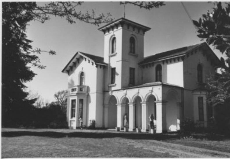
Figure 8. 'Northbury' of 1862, Longford, Tasmania (source: National Trust of Tasmania, 1965)
