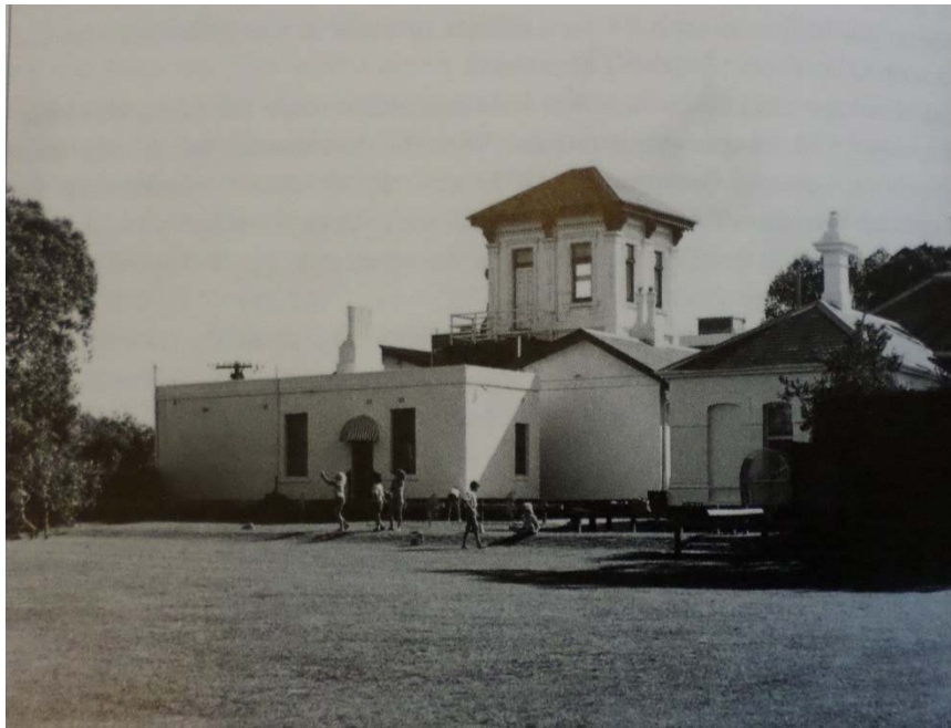
Figure 3. 'The Pottery' at Glamorgan, photographed after demolition of the coach house and renovations in 1978 (source: Andrew Lemon, The Pride of Miss McComas , 1993).
