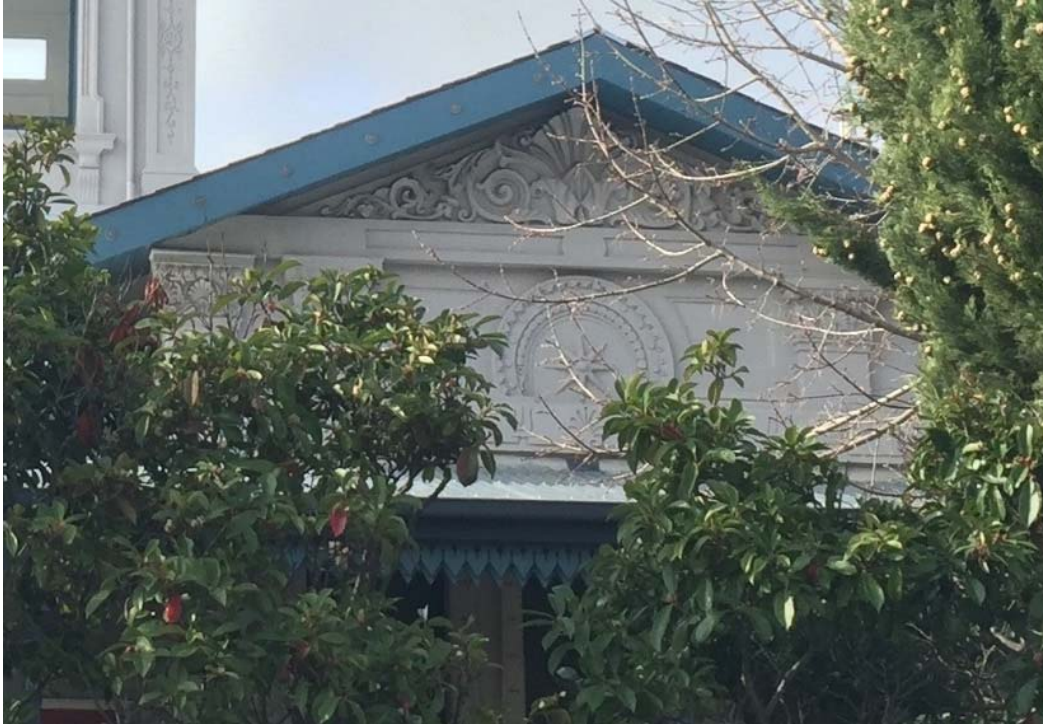
Figure 6. Detail of the elaborate high relief render tympanum to the front projecting bay. The scalloped fringe to the verandah is just visible below (source: City of Stonnington 2016).
