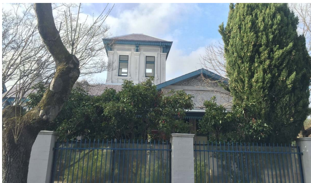
Figure 5. Front elevation of 'Hybla' (source: City of Stonnington 2016).
