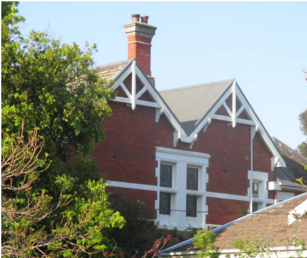
Figure 4. First floor of the south elevation showing a chimney, the decorative gable trusses, red brick and window configuration (source: Context 2016).
