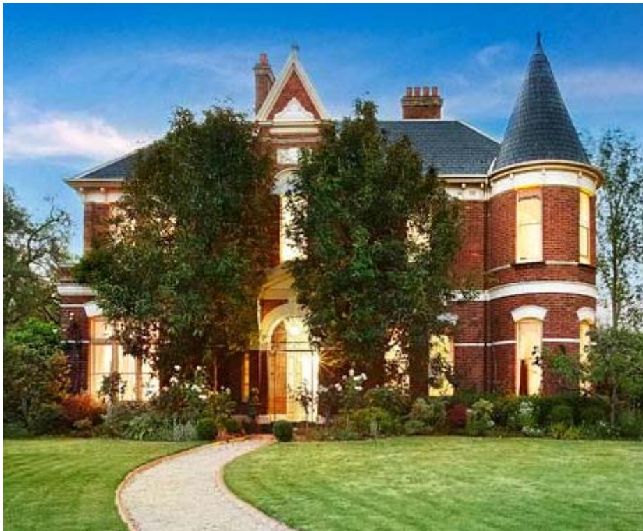
Figure 7. 59 Kensington Road, South Yarra (HO64) (source: R.T. Edgar 2010).
