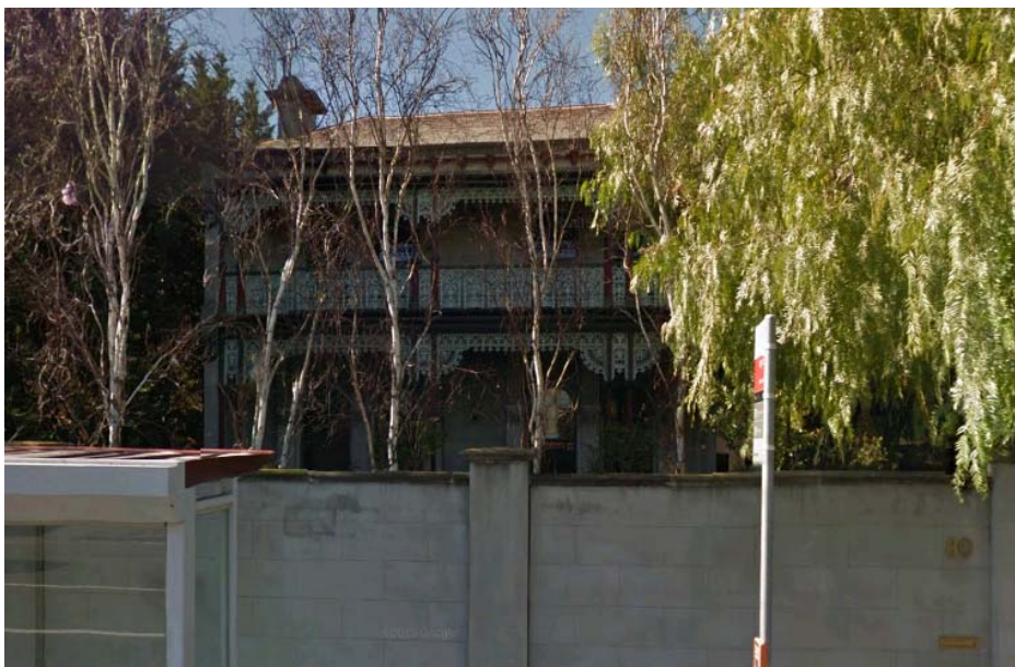
Figure 7. 80 Williams Road, Prahran, significant in HO155 (source: Google Streetview).
