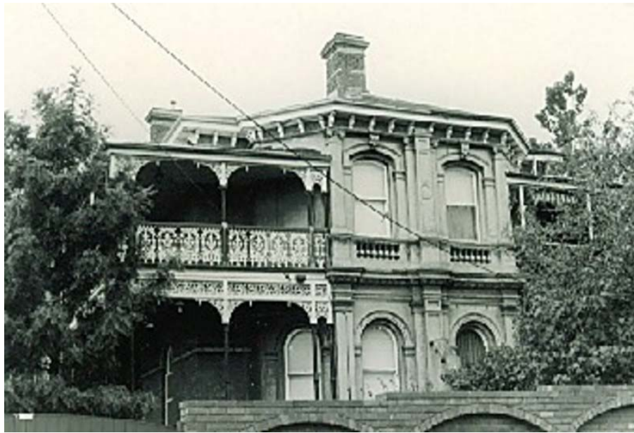
Figure 2. 14 & 16 William Street, South Yarra. Note: the original balustrade cast-iron to no. 16 is visible here. (source: National Trust file B4391)
