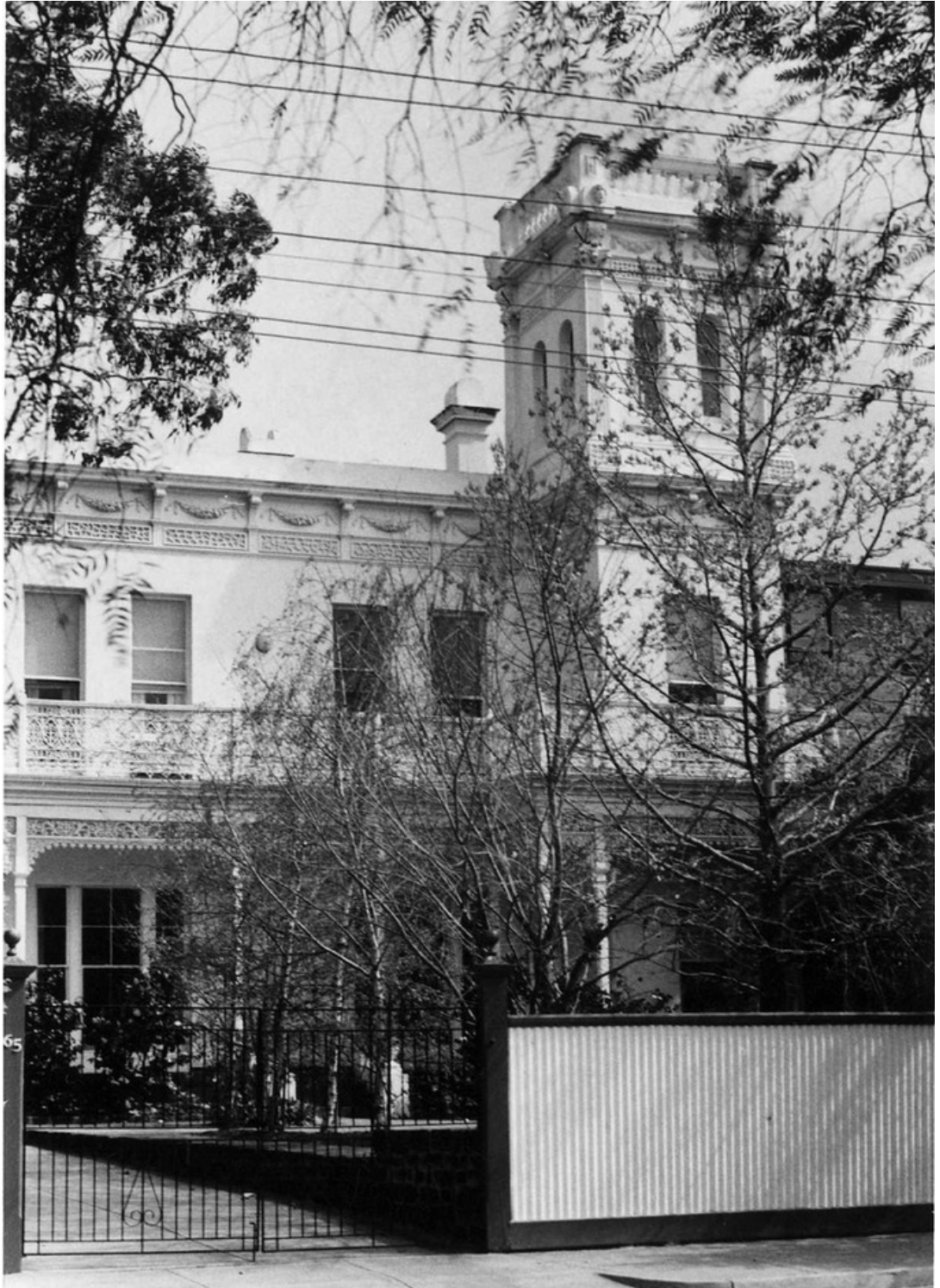
Figure 2. 65 Murphy Street in the late 1960s (source: John Collins Collection, SLV)
