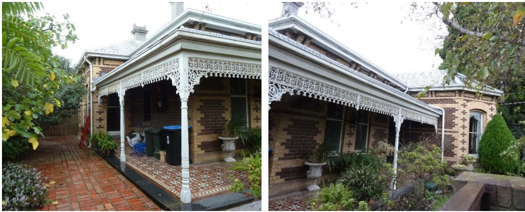
Figure 4. Front and side elevations of 25 Winter Street, Malvern showing elaborate bichrome brick patterning (source: Context 2016).
