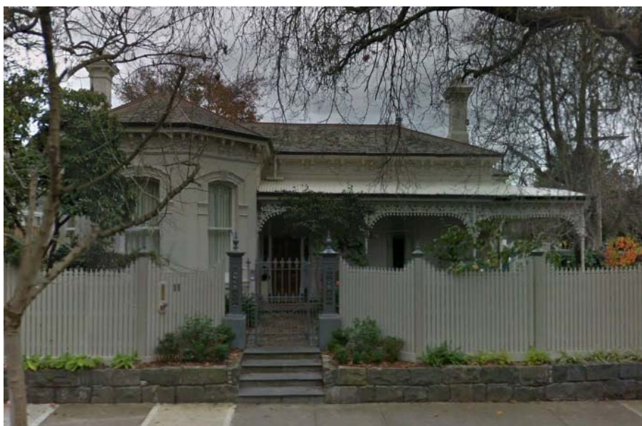
Figure 6. 11 Avondale Road, Armadale, individually significant in HO123 (source: Google Streetview).
