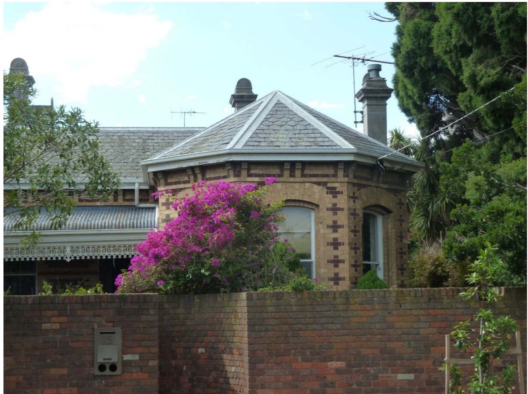
Figure 5. Front elevation of canted bay as seen from Winter Street (source: Context 2016).
