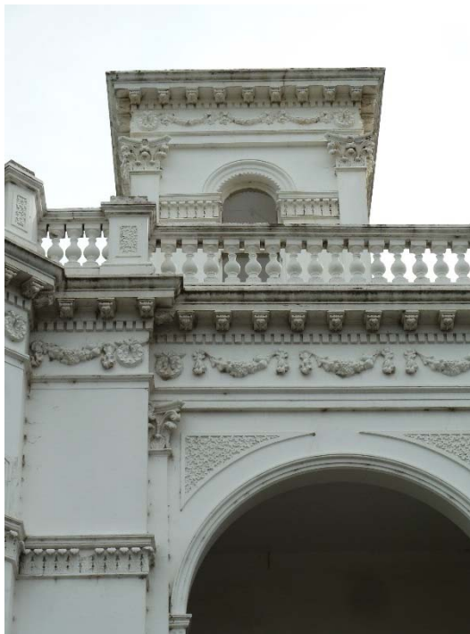
Figure 4. Detail of Classical detailing including the balustraded parapet and central tower (source: Context 2016).
