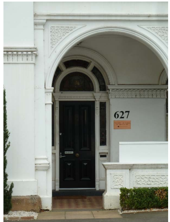
Figure 5. Detail of the highly intact and elaborate front door (source: Context 2016).
