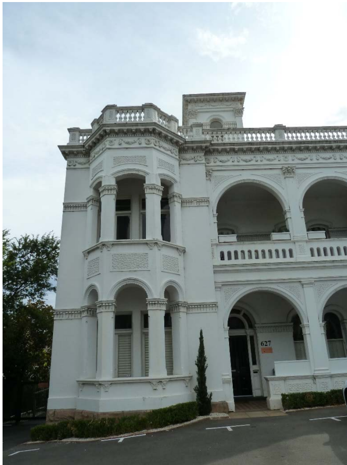
Figure 3. Detail of canted masonry loggia to the projecting bay fronting Malvern Road (source: Context 2016).
