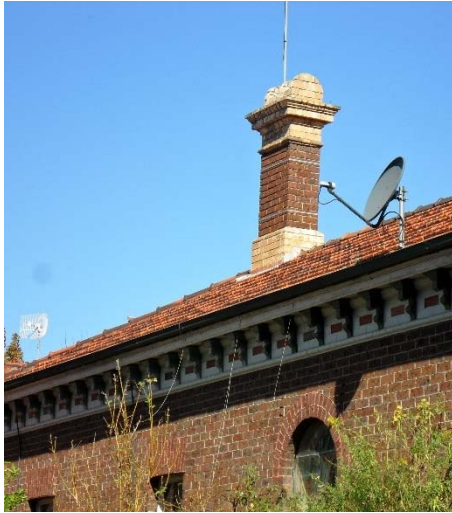
Figure 5. Detail of unusual brick wythes to the bichrome brick chimneys (source: Context 2016).
