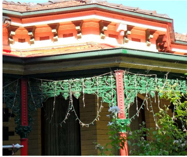
Figure 6. Detail of intact cast-iron verandah (source: Context 2016).
