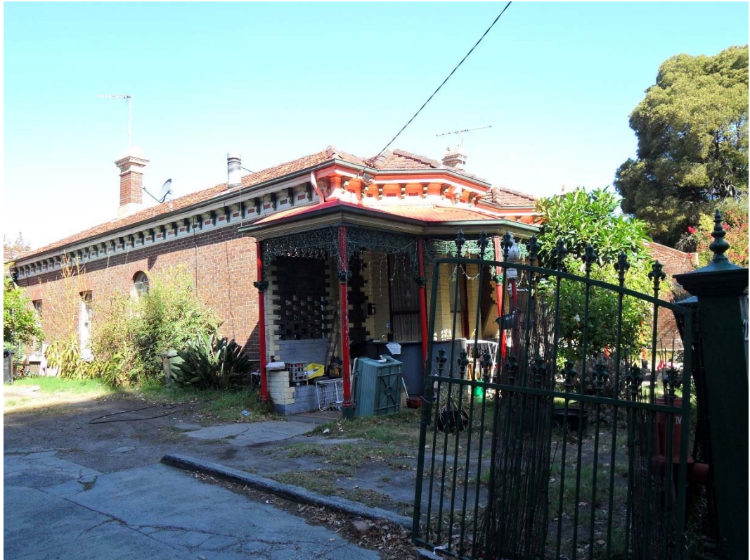
Figure 4. View of front elevation, looking south-east (source: Context 2016).
