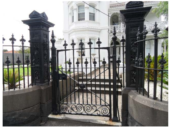
Figure 4. Detail of pedestrian gate to iron palisade fence (source: Context 2016).
