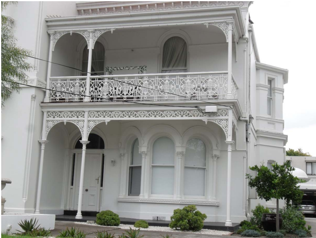
Figure 5. Detail of two storey cast iron verandah with canted bay window to the ground level (source: Context 2016).
