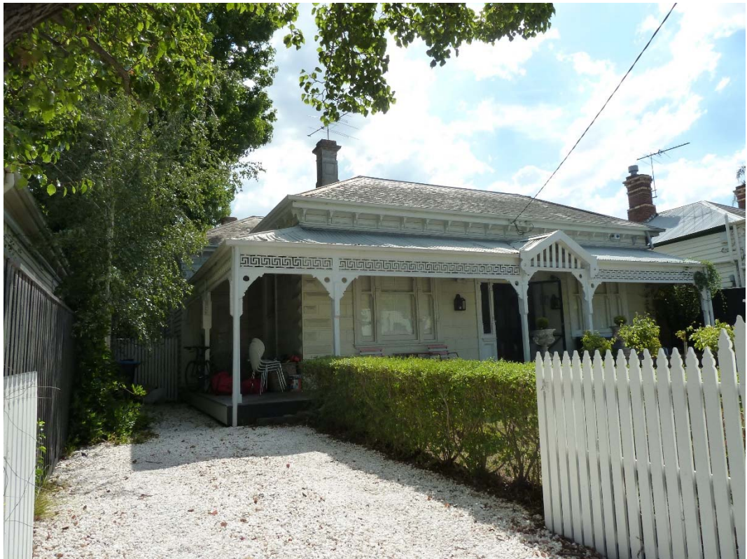
Figure 3. View looking north-east showing the return verandah (source: Context 2016).
