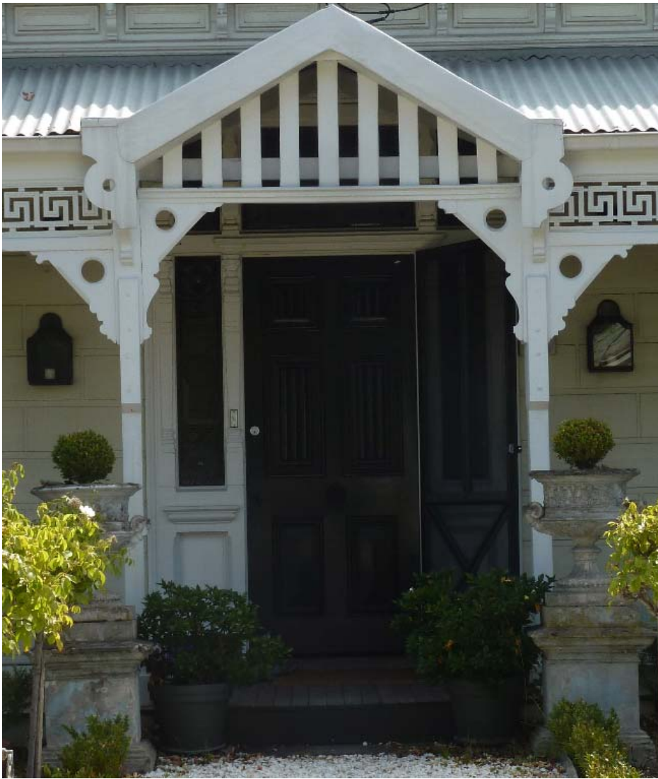
Figure 2. View of entrance detail (source: Context 2016).
