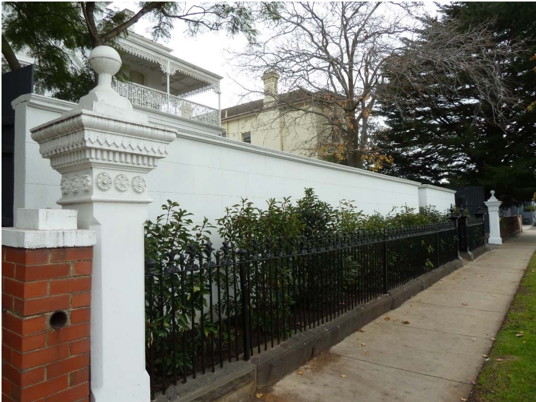
Figure 5. Detail of the iron palisade fence with highly decorative masonry piers that has been retained in front of a new masonry front wall (source: Context 2016).
