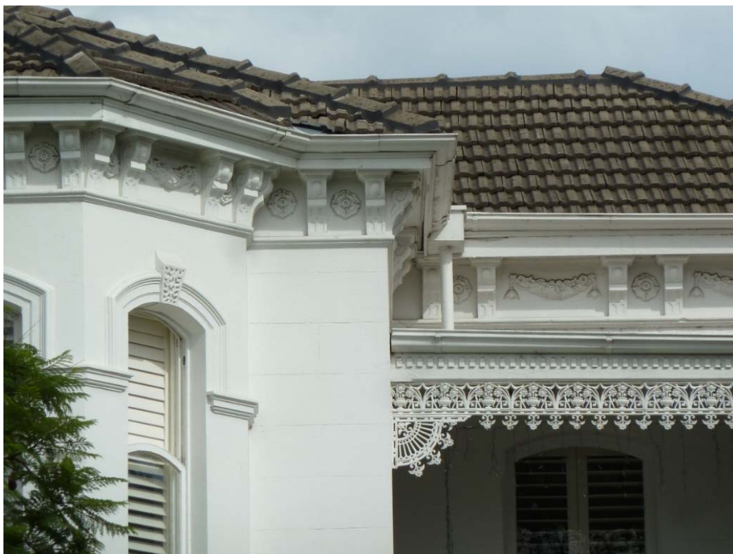
Figure 4. Detail of 173 Tooronga Road, Glen Iris (source: Context 2016).
