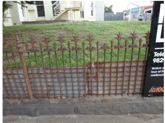
Figure 9. Iron palisade fence with corrugated iron retaining on a bluestone plinth at no. 175 Tooronga Road, Glen Iris (Context 2016).
