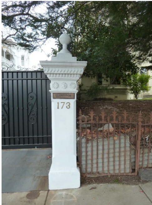
Figure 8. Detail of masonry pier to no. 173 Tooronga Road, Glen Iris and neighbouring iron palisade fence with bluestone plinth to no. 175 Tooronga Road, Glen Iris (source: Context 2016).
