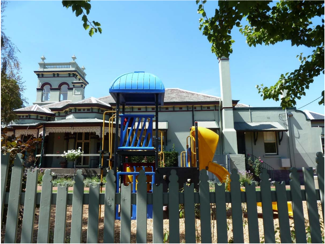
Figure 9. West elevation of 'Blairholme' showing the later extensions to the rear (south) (source: Context 2016).
