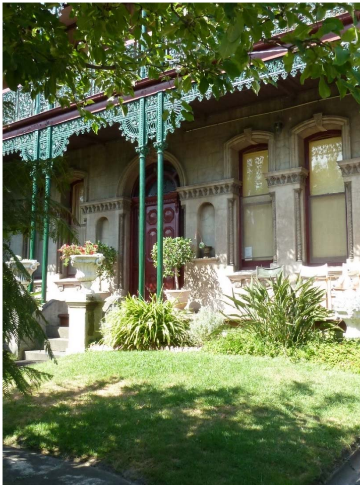
Figure 4. Detail of impressive cast and run cement render details to ground floor and elaborate front door composition (source: Context 2016).
