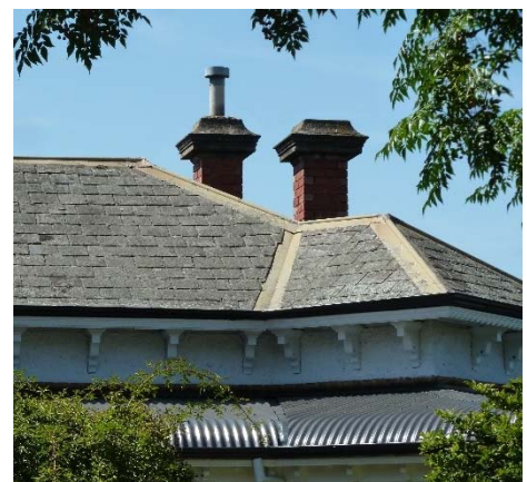
Figure 6. Detail of complex slate clad roof with red brick chimneys with heavy unpainted cement cornices (source: Context 2016).
