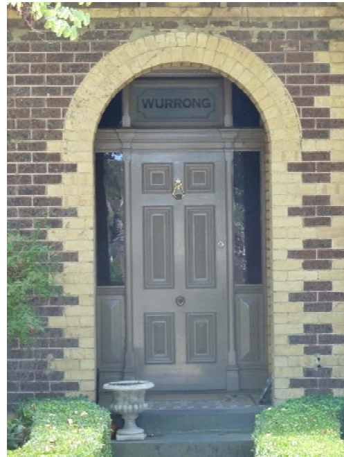
Figure 4. Detail of front entrance door (source: Context 2016).
