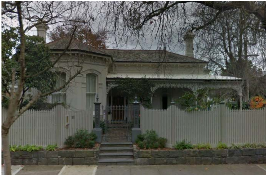
Figure 5. 11 Avondale Road, Armadale, individually significant in HO123 (source: Google Streetview).
