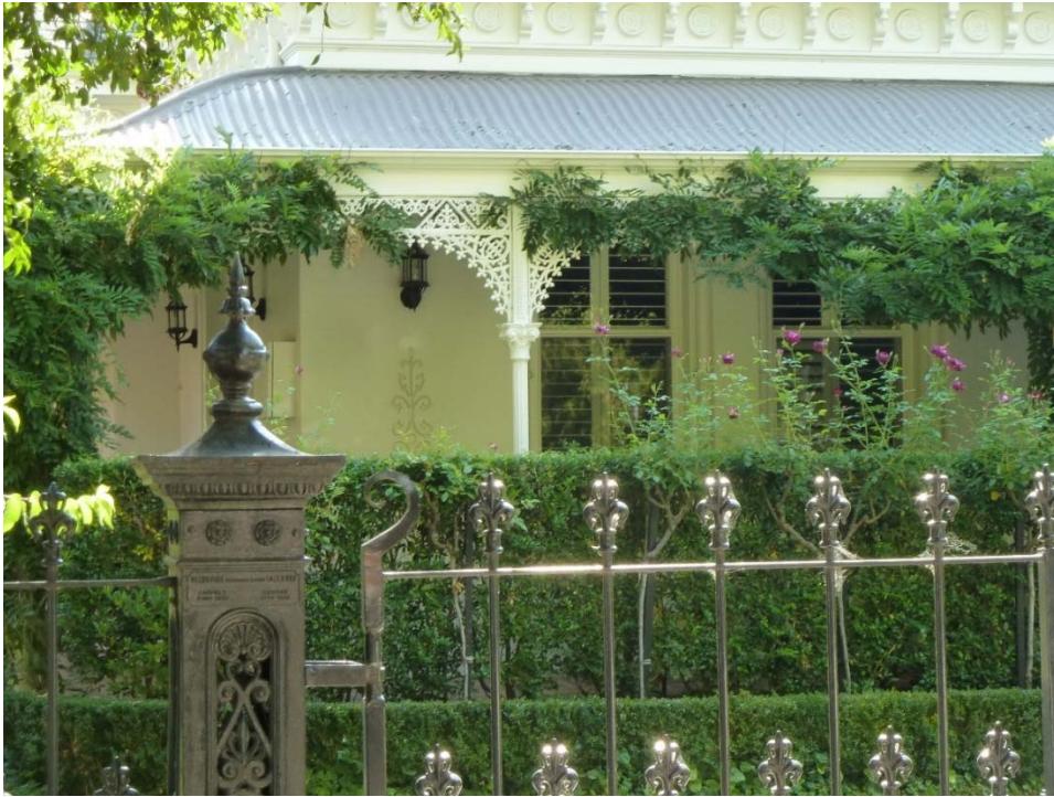
Figure 2. Detail of fine incised floral patterns to the render and cast iron ogee verandah. The palisade fence in the foreground is a sympathetic reproduction (source: Context 2016)
