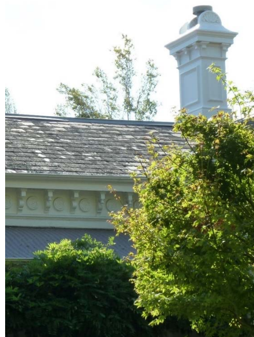
Figure 4. Detail showing render details to chimney and cornice with eaves brackets (source: Context 2016)
