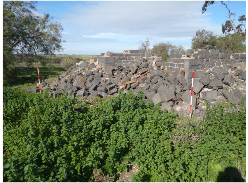
View southeast of walls on east side of ruin
