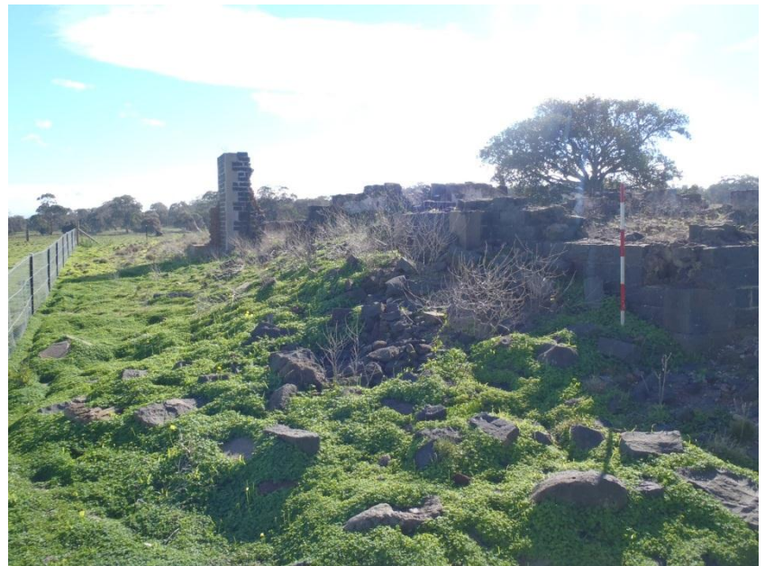
View northwest of walls along the western side of the ruin
