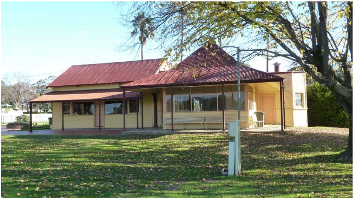
The east elevation of Lienhop Lodge.
