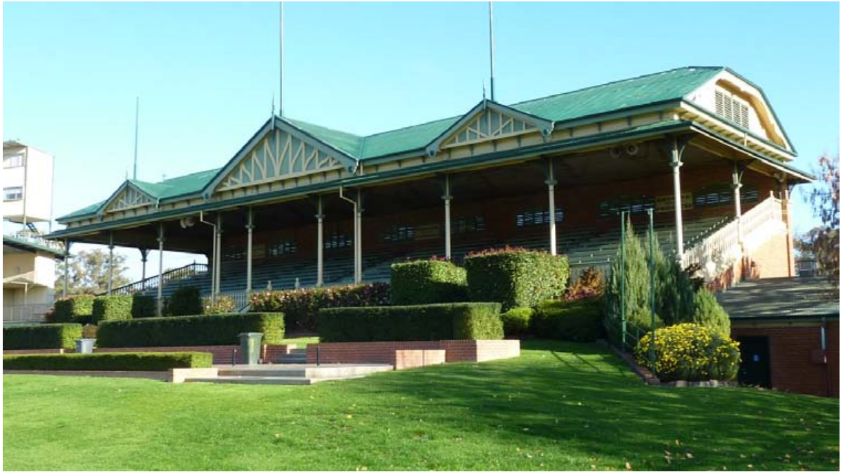
The 1902 Grandstand as viewed from the east.
