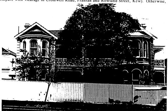
they are of more typical nineteenth century Italianate form with respect to their projecting bay windows and restrained classical derived detailing. These buildings are substantially intact other than the slate roof being replaced with terracotta tiles, the loss of finial to No 29 and the complete removal of the original gable end detailing at No 27 and the virtual removal of the side verandah at No 27. The front fences are also of a later relatively unsympathetic character.
