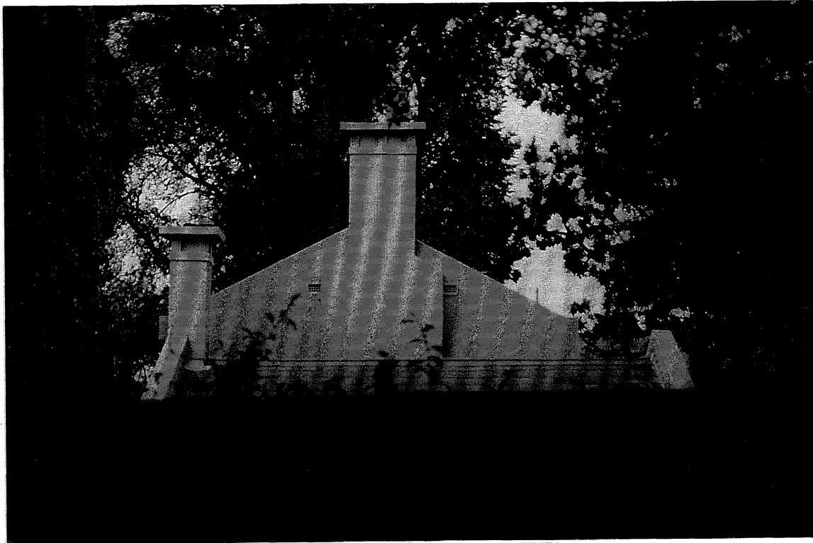
View from Albany Road showing Butler chimney design, and gable parapet, 1920 single storey extension in foreground
