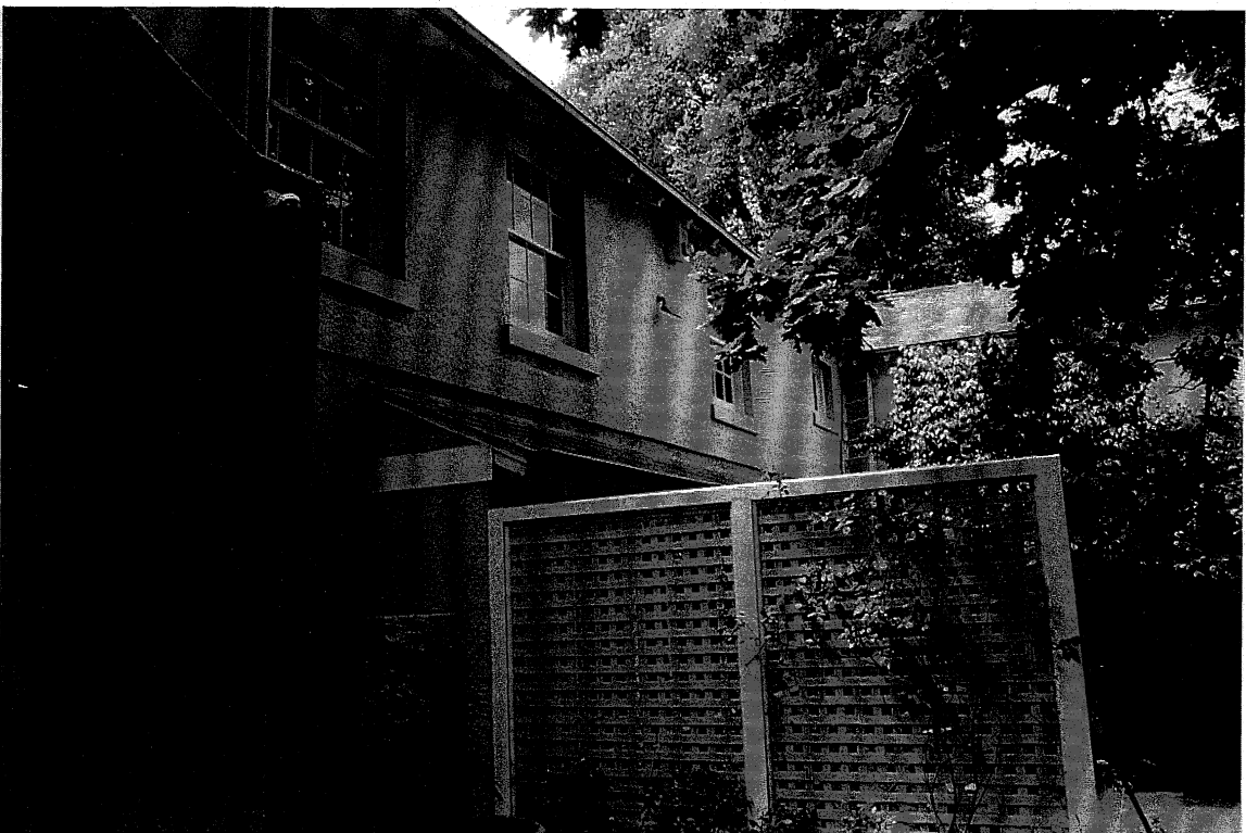
View along side elevation, showing single storey extension for enlarged motor garage, and second storey extension over former laundry
