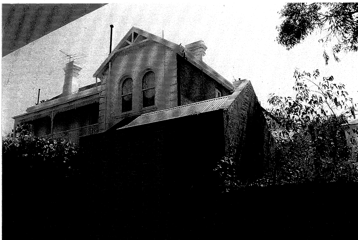
Rear view of number 29, showing rear of other house facing Kooyong Road shown in MMBW plan
