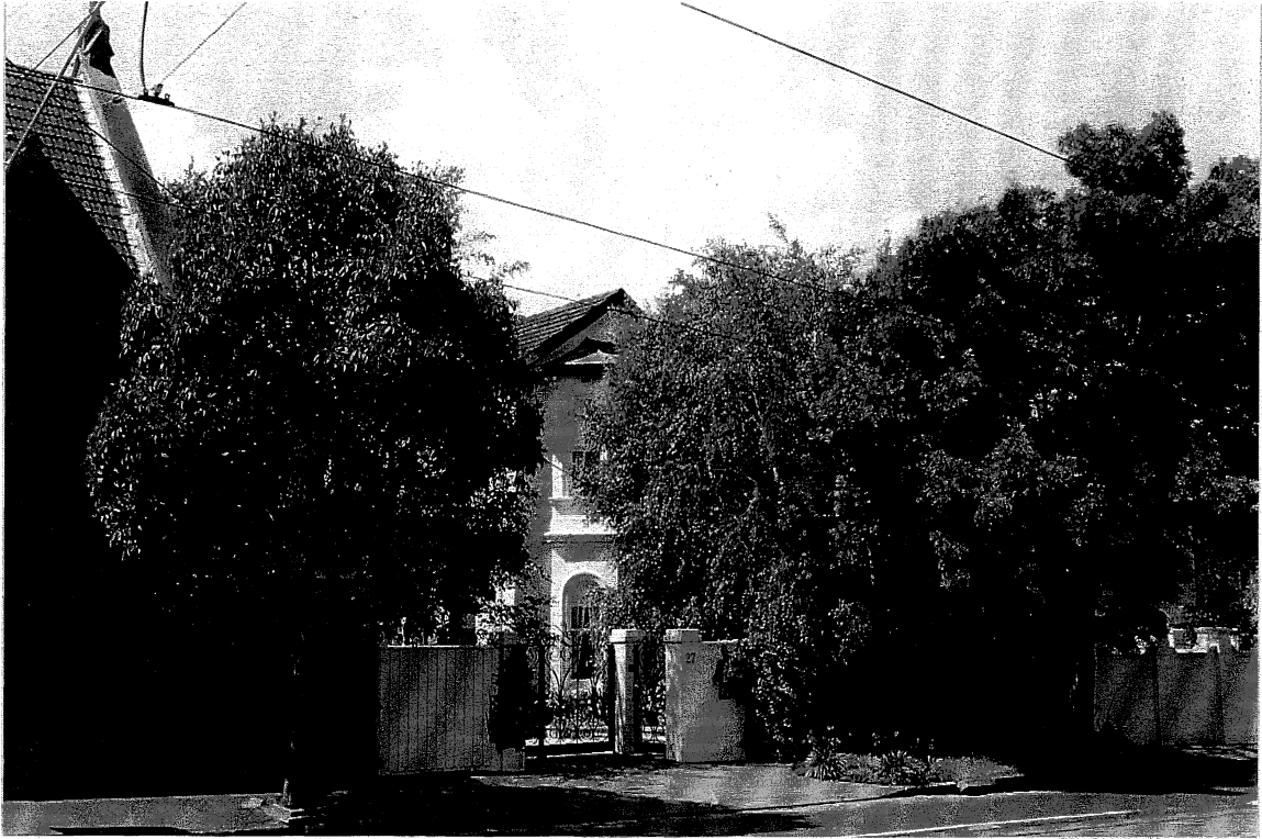
Number 27 (former vicarage) and former church hall
