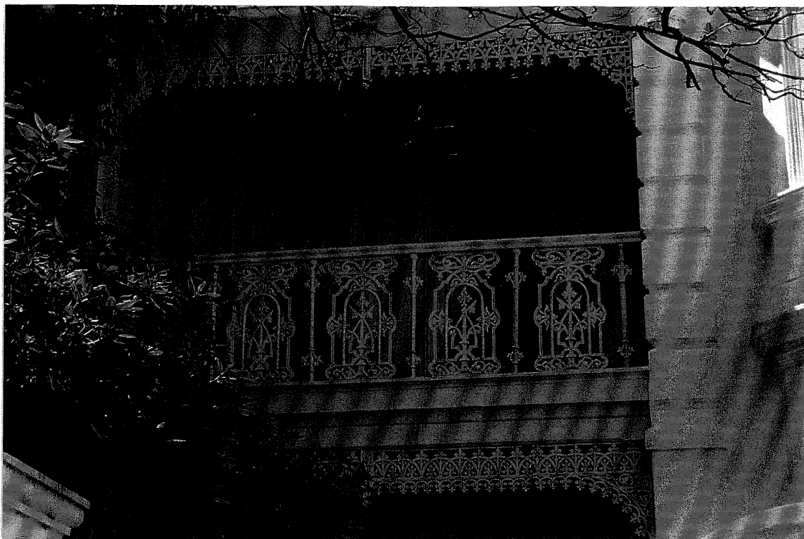
Detail of front verandah of number 29, and converted windows
