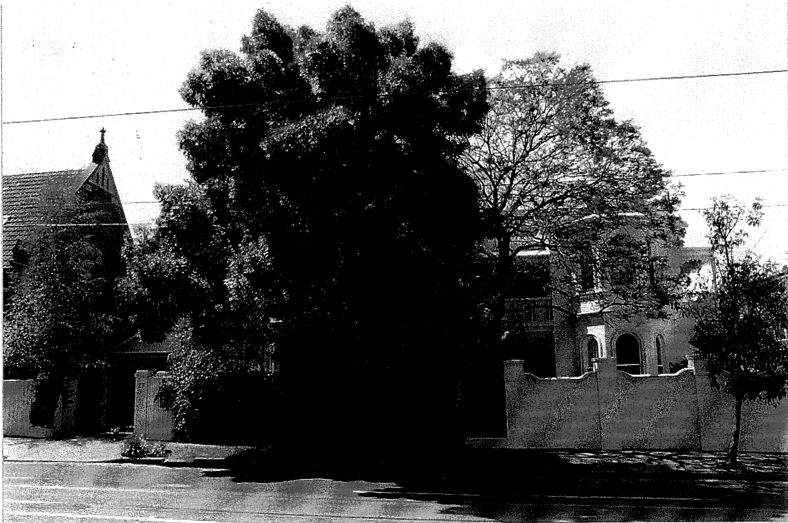
View from cross road showing former church hall
