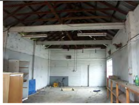
Photo 3.64: Former Sloyd Room (Building 7), interior of front (northern) portion.
