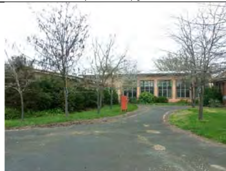
Photo 3.66: East façade of the northern wing of the former Service Block, Dining Room & Intermediate Cottage (Building 9).
