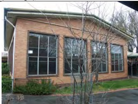
Photo 3.65: North façade of the northern wing of the former Service Block, Dining Room & Intermediate Cottage (Building 9).
