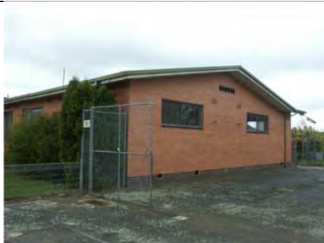
Photo 3.57: Former Albert Leach Cottage (Building 5), west elevation.
