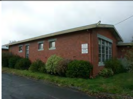
Photo 3.41: Former School (Building 4), north elevation of north wing.
