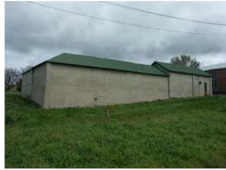
Photo 3.62: Former Sloyd Room & Stores (Building 7): east elevation.
