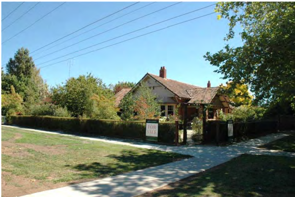
Photo 4.16: Dwelling, 101 Forrest Street, Ballarat, 2005. Source: D. Rowe & W. Jacobs, Ballarat Precincts Study, prepared for the City of Ballarat, 2005.
