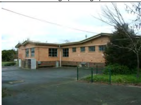
Photo 3.67: East façade of the east wing of the former Service Block, Dining Room & Intermediate Cottage (Building 9).
