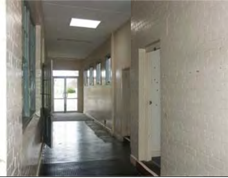
Photo 3.54: Former School (Building 4), interior of rear corridor (infilled verandah).
