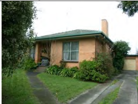
Photo 3.81: Former Superintendent's Residence (Building 10).
