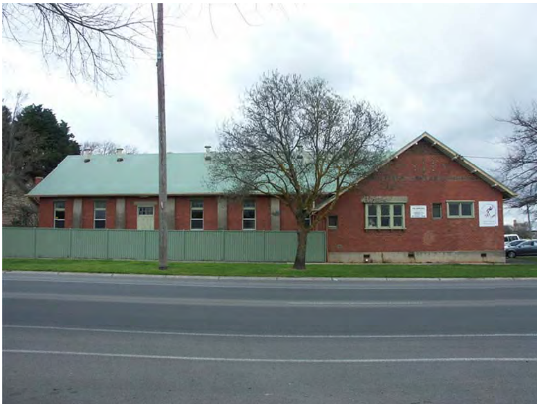
Photo 4.18: Former Ballarat North Progress Association Hall, 820 Armstrong Street North, Ballarat, 2011. Source: David Rowe.
