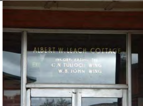
Photo 3.58: Former Albert Leach Cottage (Building 5), detail of transom above main entry.
