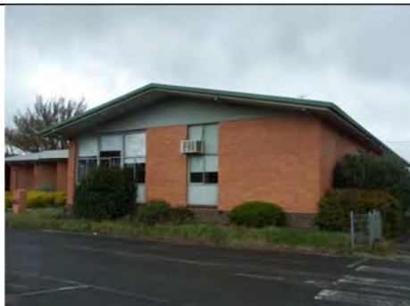
Photo 3.35: Former William Farrell Cottage (Building 3), north elevation of projecting front gable.
