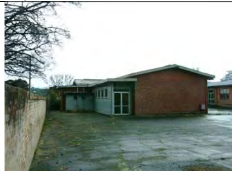
Photo 3.44: Former School (Building 4), south elevation.
