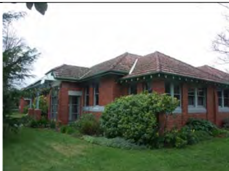
Photo 3.17: Former Toddlers' Block (Building 1), north-west corner.
