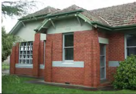
Photo 3.21: Former Toddlers' Block (Building 1), north elevation of north-eastern portion of the James Kerslake wing added in 1939.
