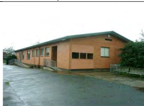
Photo 3.36: Former William Farrell Cottage (Building 3), south elevation (west portion).
