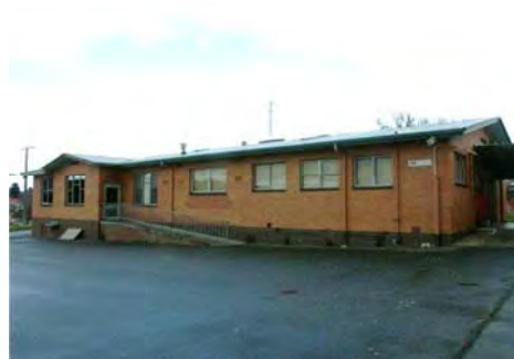
Photo 3.60: Former Albert Leach Cottage (Building 6), east elevation.
