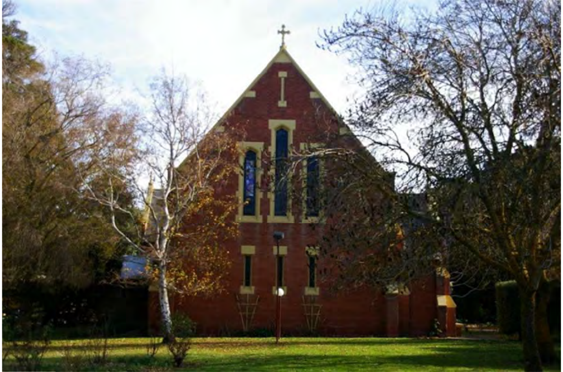
Photo 4.09: Former St. Joseph's Orphanage Chapel, Grant Street, Sebastopol, 2011. Source: Heritage Victoria (HERMES).
