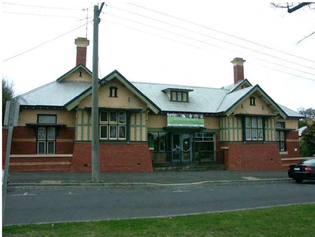
Figure 2.52: Former Boy's Hostel, Victoria Street, Ballarat, August 2011. Source: David Rowe.
