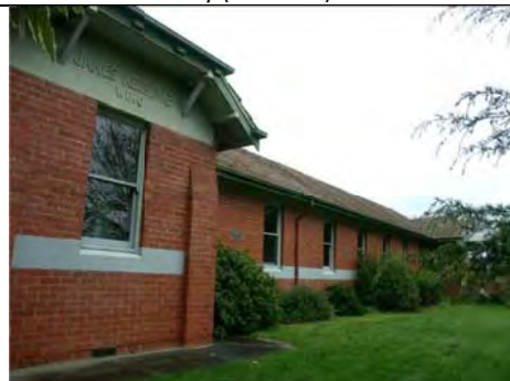
Photo 3.18: Former Toddlers' Block (Building 1) north elevation, east end (looking west).
