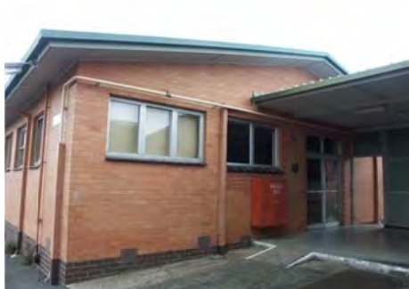
Photo 3.59: Former Albert Leach Cottage (Building 5), south addition showing flat-roofed link to Building 6.
