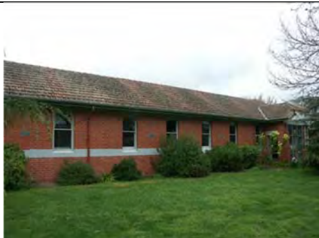
Photo 3.19: Former Toddlers' Block (Building 1), central portion of north elevation.
