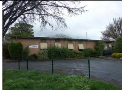
Photo 3.32: Former Administration Block (Building 2), west elevation.
