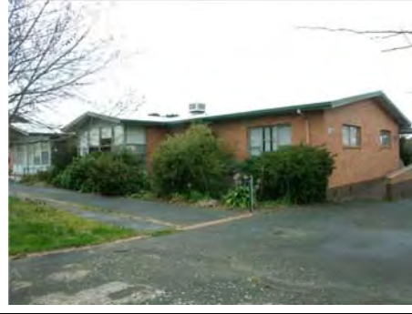
Photo 3.76: Former Bluebird's Cottage (Building 9), north elevation.
