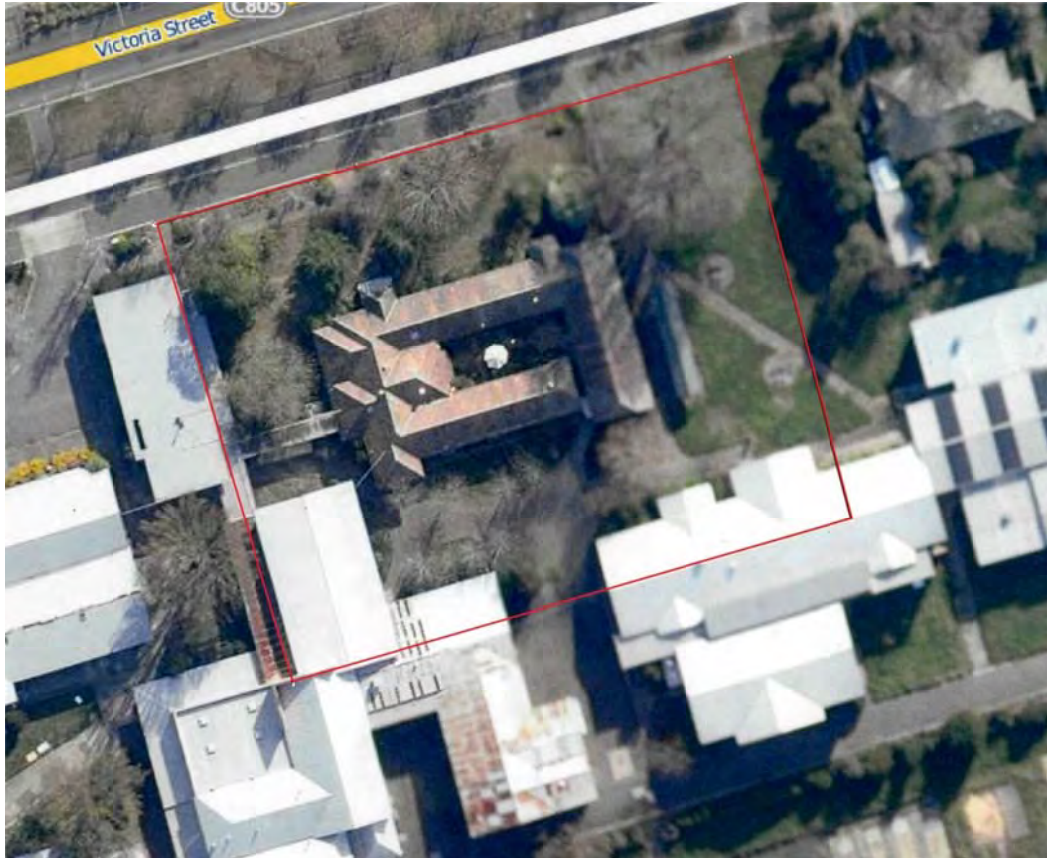
Detailed Aerial Image showing potential extent of the individual heritage overlay. Source: NearMaps.
