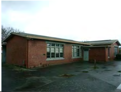
Photo 3.45: Former School (Building 4), east elevation.
