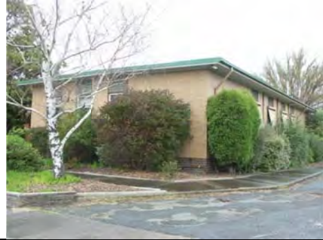
Photo 3.30: Former Administration Block (Building 2), north and west elevations.
