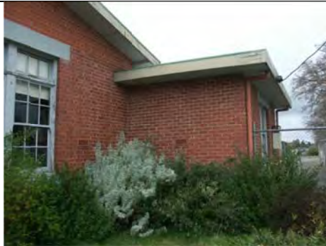
Photo 3.47: Former School (Building 4), north elevation of projecting minor west wing.
