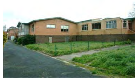
Photo 3.78: Former Bluebird's Cottage, south elevation (east end) showing parapeted addition.
