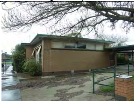
Photo 3.33: Former Administration Block (Building 2), south elevation.
