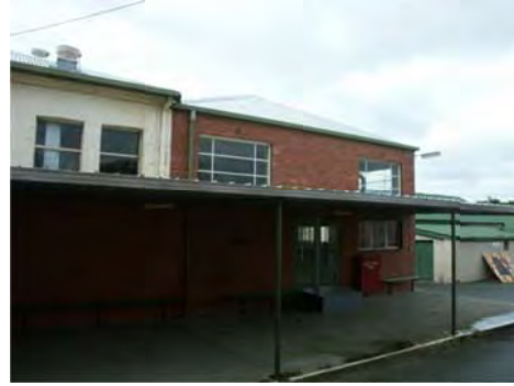
Photo 3.74: Former Gymnasium addition (built 1952), west elevation, Building 9.
