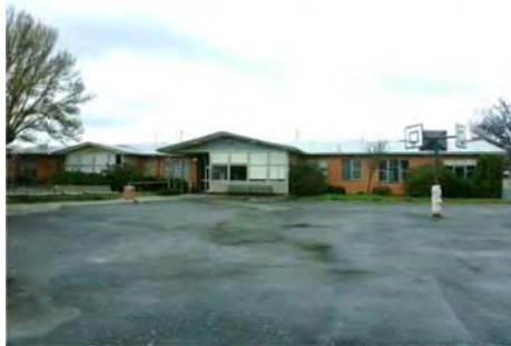
Photo 3.55: Former Albert Leach Cottage (Building 5), north elevation.
