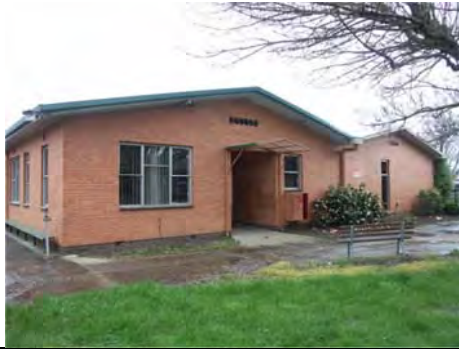
Photo 3.37: Former William Farrell Cottage (Building 3), east elevation (the northern[right] gable reflects the addition of 1999).
