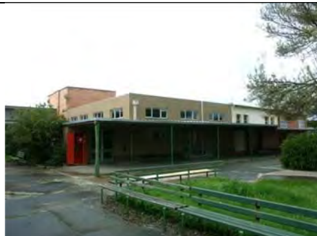
Photo 3.71: North-west wing (later addition in the location of the former swimming pool), Building 9.
