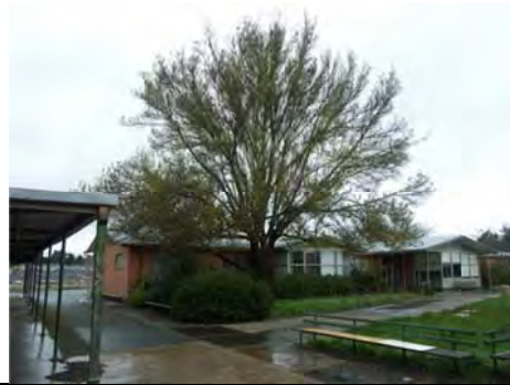
Photo 3.14: Landscaped area south of the former William Farrell Cottage (building 3).
