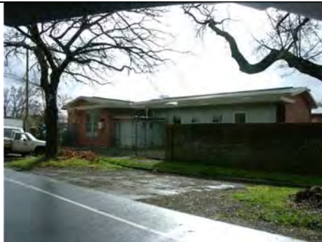
Photo 3.43: Former School (Building 4), west elevation showing infilled verandah and introduced toilet wing.
