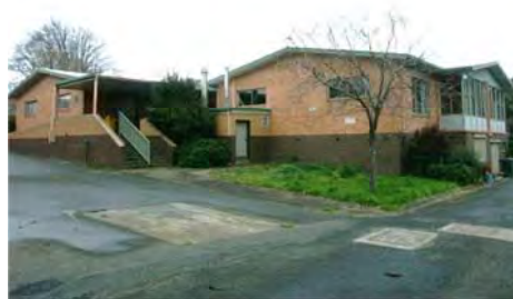
Photo 3.77: Former Bluebird's Cottage (Building 9), west elevation.
