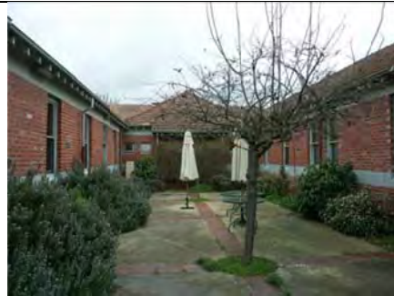
Photo 3.24: Former Toddlers' Block (Building 1), courtyard looking west.
