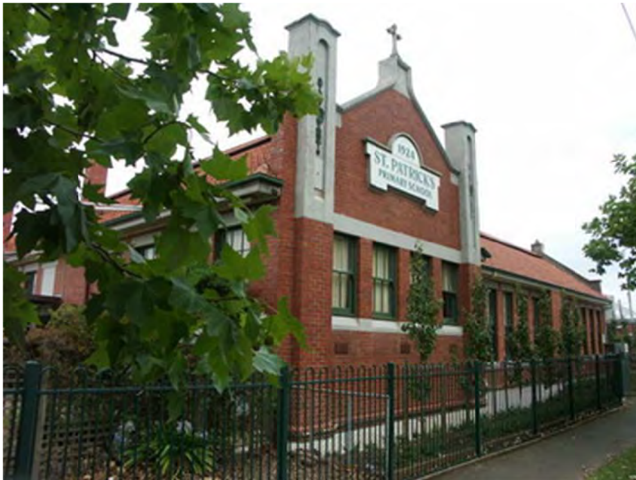
Photo 4.22: St. Patrick's Primary School, Drummond Street South, Ballarat, 2007. Source: David Rowe.
