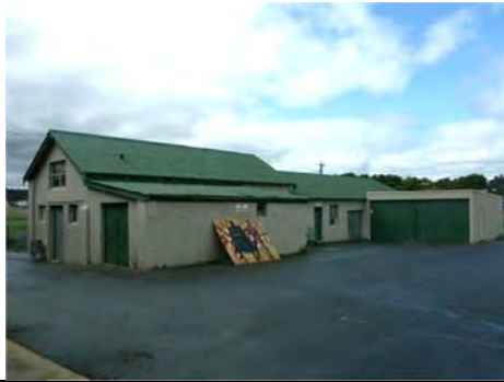
Photo 3.61: Former Sloyd Room & Stores (Building 7): north & west elevations.
