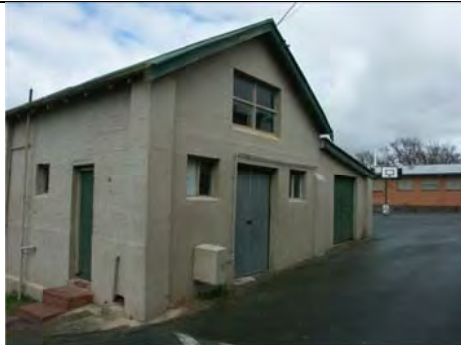
Photo 3.63: Former Sloyd Room & Stores (Building 7), north elevation.
