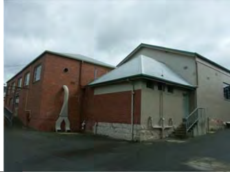
Photo 3.75: Former Gymnasium addition (left), south elevation, Building 9.
