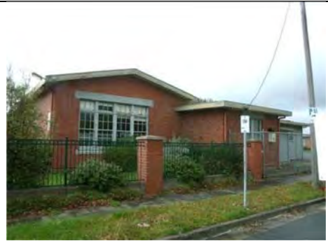
Photo 3.42: Former School (Building 4), west elevation of north wing and projecting minor wing.
