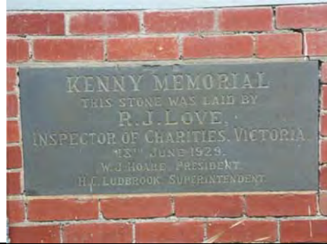
Photo 3.22: Former Toddlers' Block (Building 1), detail of Kenny Memorial Foundation Stone.
