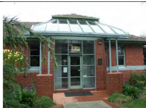
Photo 3.26: Former Toddlers' Block (Building 1), detail of front entrance with introduced glazed porch.
