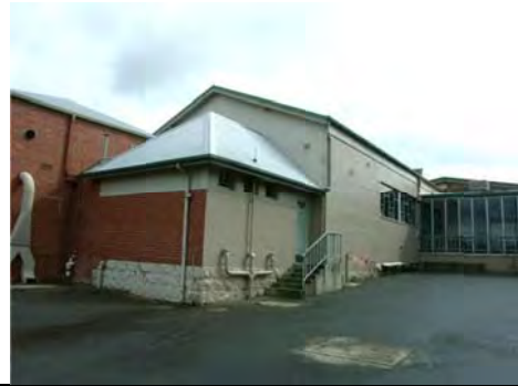
Photo 3.70: Former Gymnasium (1907 construction) & latrines wing, central section of Building 9.
