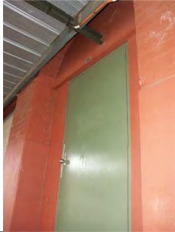
Photo 3.73: Round arched opening detail, west façade, former picture theatre wing, Building 9.
