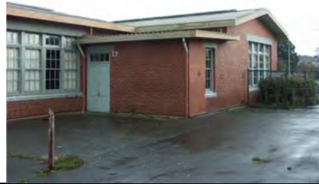
Photo 3.46: Former School (Building 4), east and south elevations of entrance wing.
