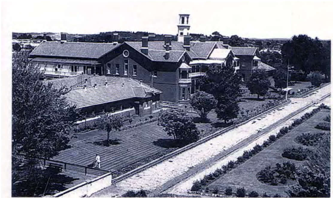
Figure 2.39: View of the Victoria Street frontage of the Ballarat Orphanage (eastern end), 1957, showing the lawned area outside the Toddlers' Block. Source: Annual Report, 1957.
