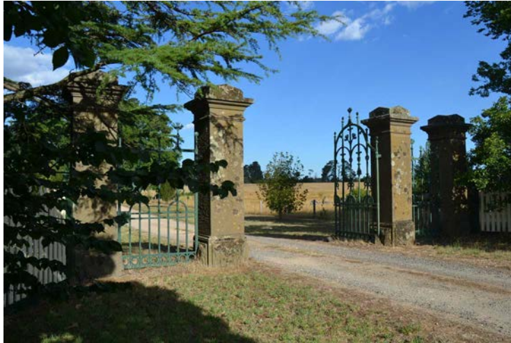
Photo 1 Gate posts and cast iron gates
