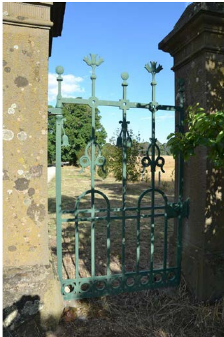
Photo 2 Detail of pedestrian gate
