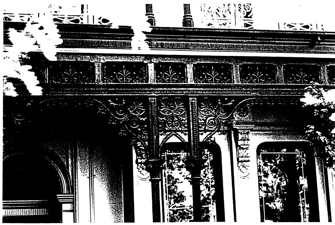
Illustration 1 Detail of cast iron and stucco work, 13 Cromwell Road, 1998. Source: Author's Collection.
