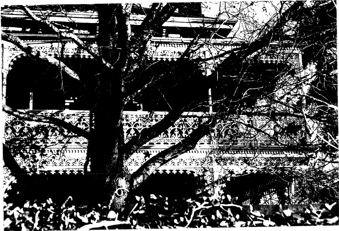
5 Detail of cast iron verandah
