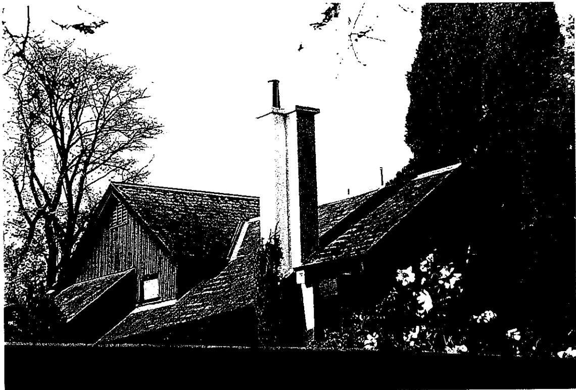
Roof of 1921 section, note chimney, roof forms, louvered vent and boarded cladding
