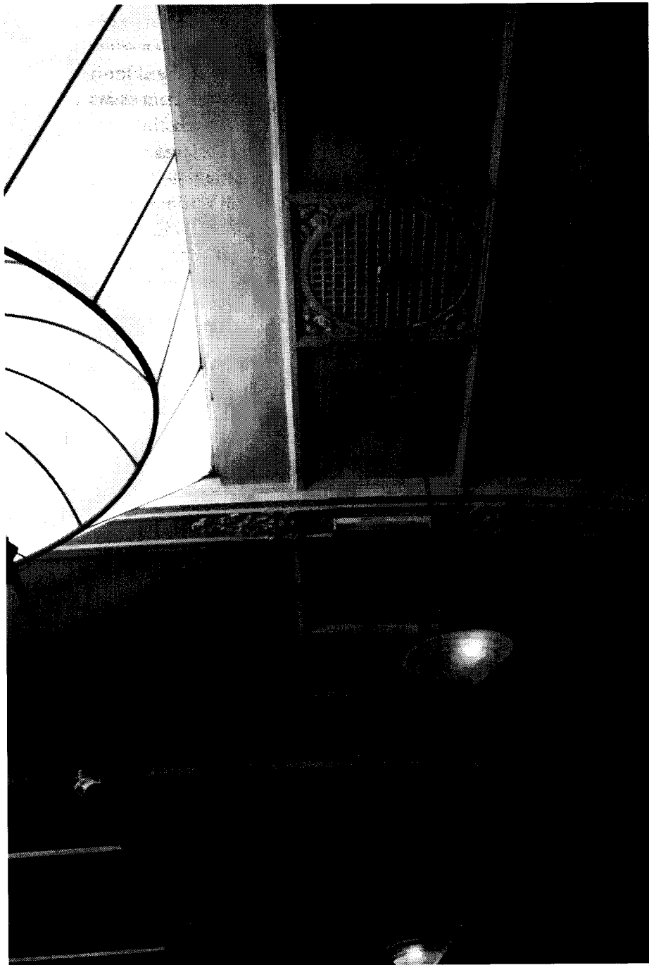
ARMADALE CINEMA – DETAIL OF BARREL CEILING & LIGHTS
