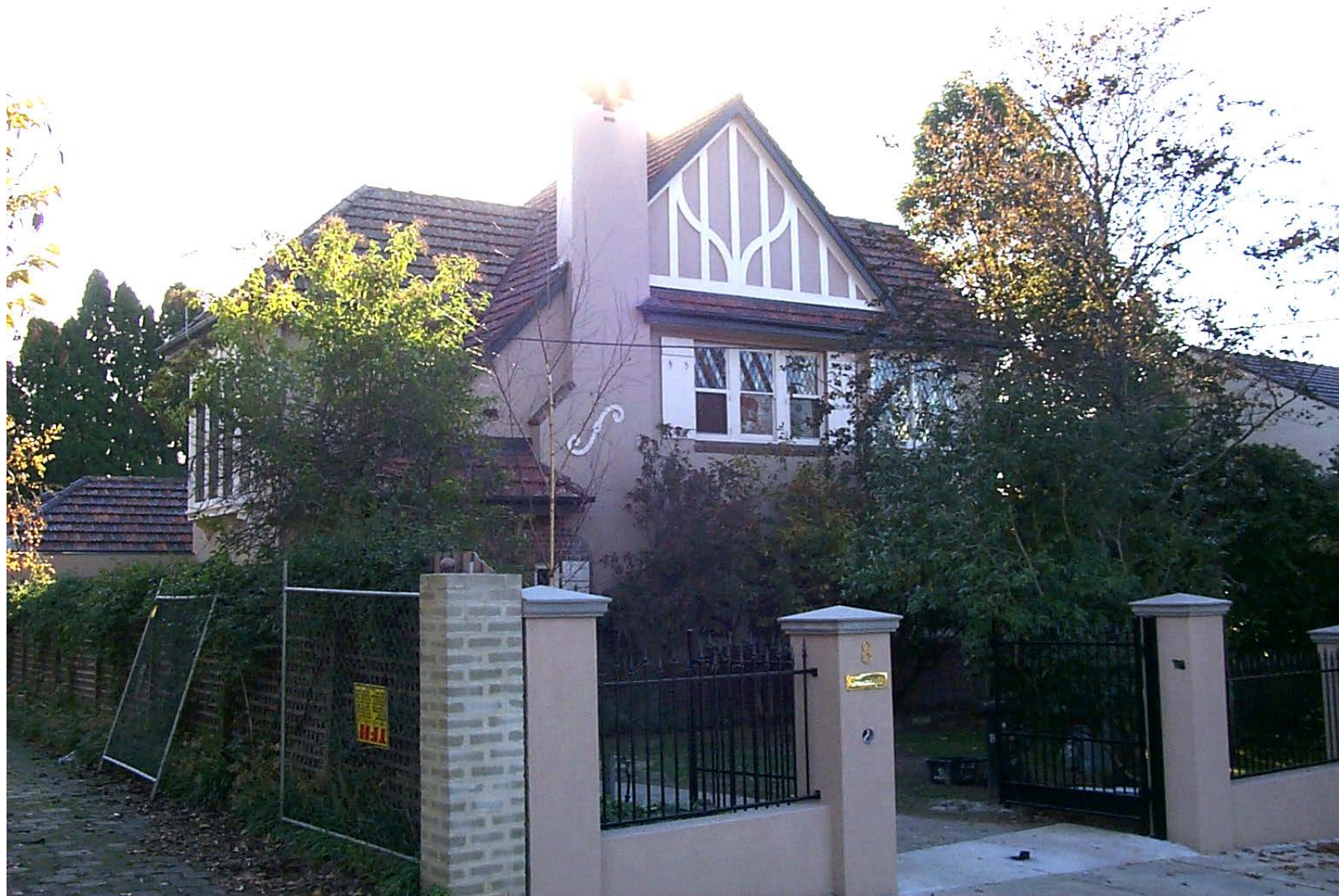
(Source: Graeme Butler & Associates May 2002 ) View from east
