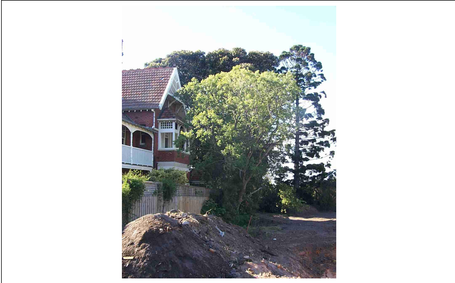
Figure 1 (Source: Graeme Butler & Associates )
