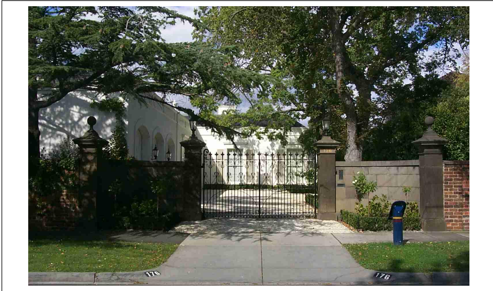
Figure 1 (Source: Graeme Butler & Associates )
