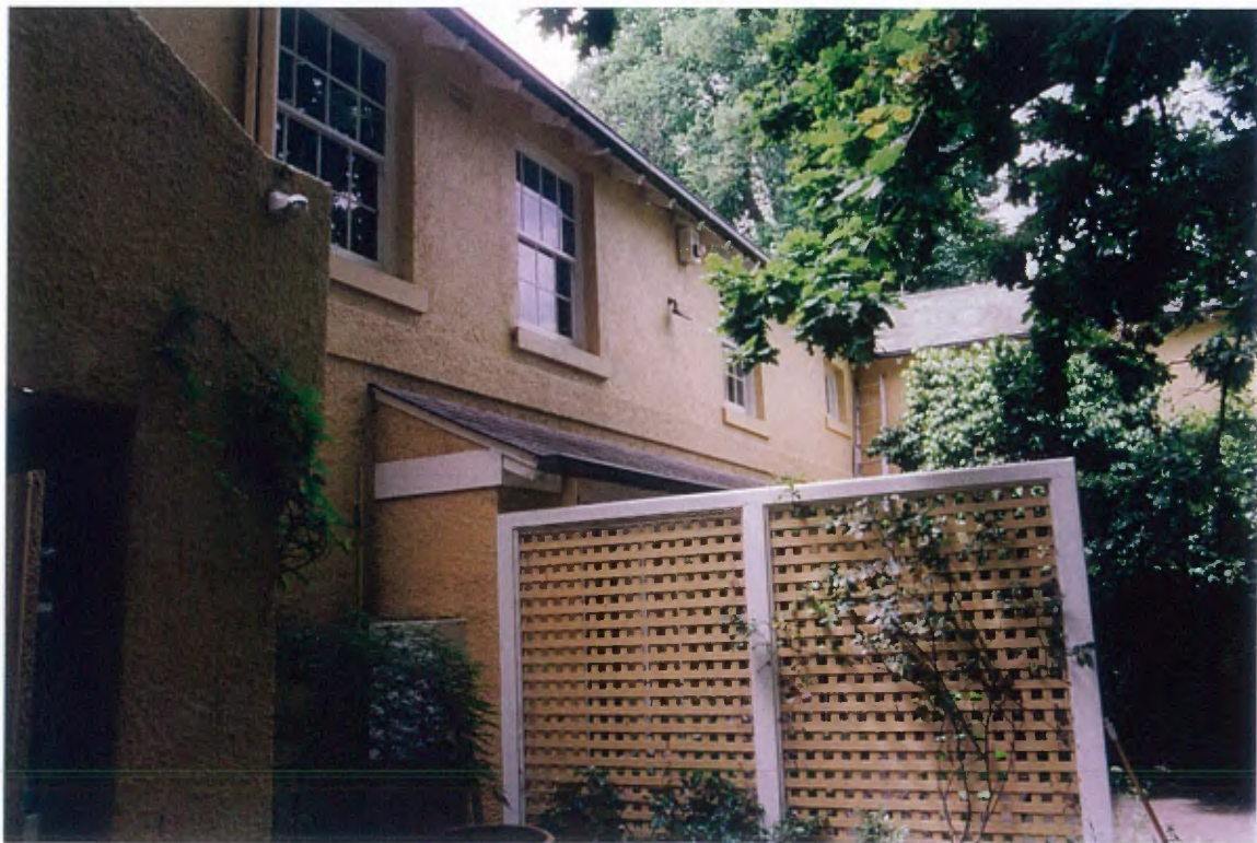
View along side elevation, showing single storey extension for enlarged motor garage, and second storey extension over former laundry
