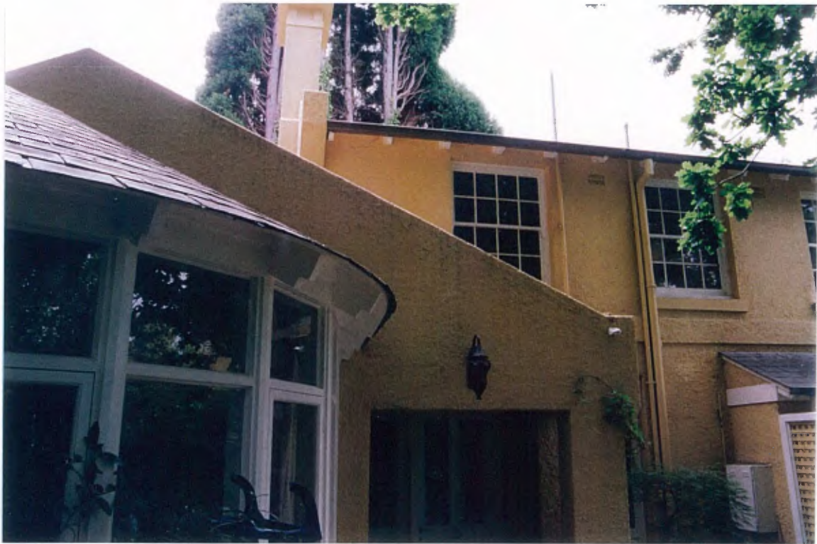
View from side of same SW section, with recent semi-circular extension in foreground
