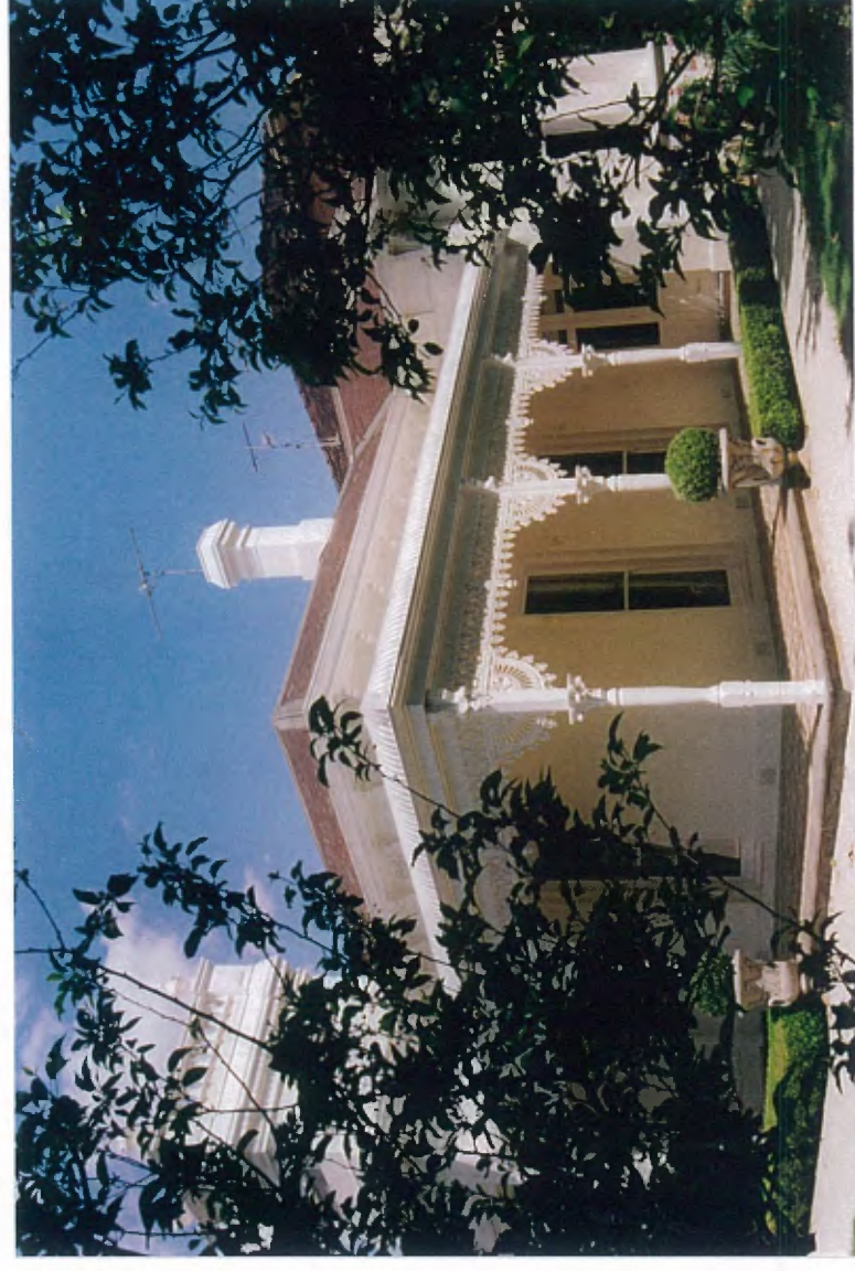
Front verandah, cast iron decoration and floor tiles
