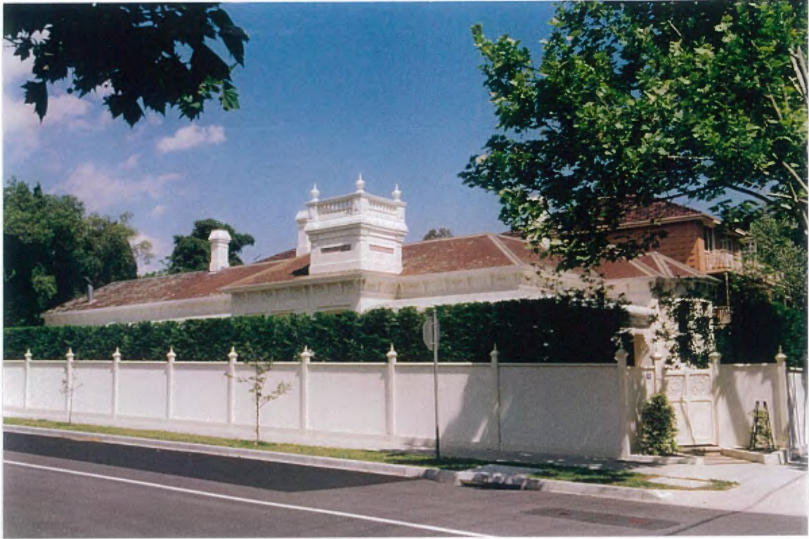
Tower and verandah relationship
