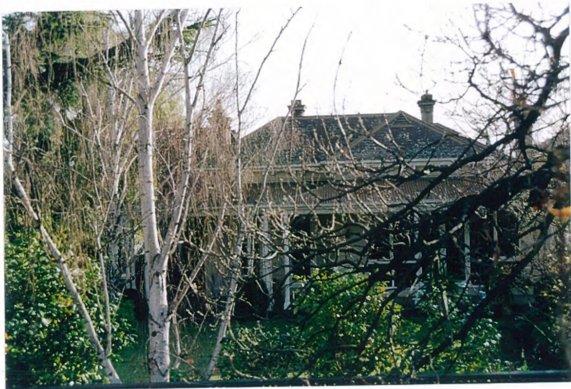
2 View of main roof form and verandah
