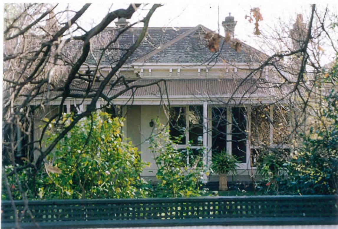
3 Detail of front verandah and altered windows
